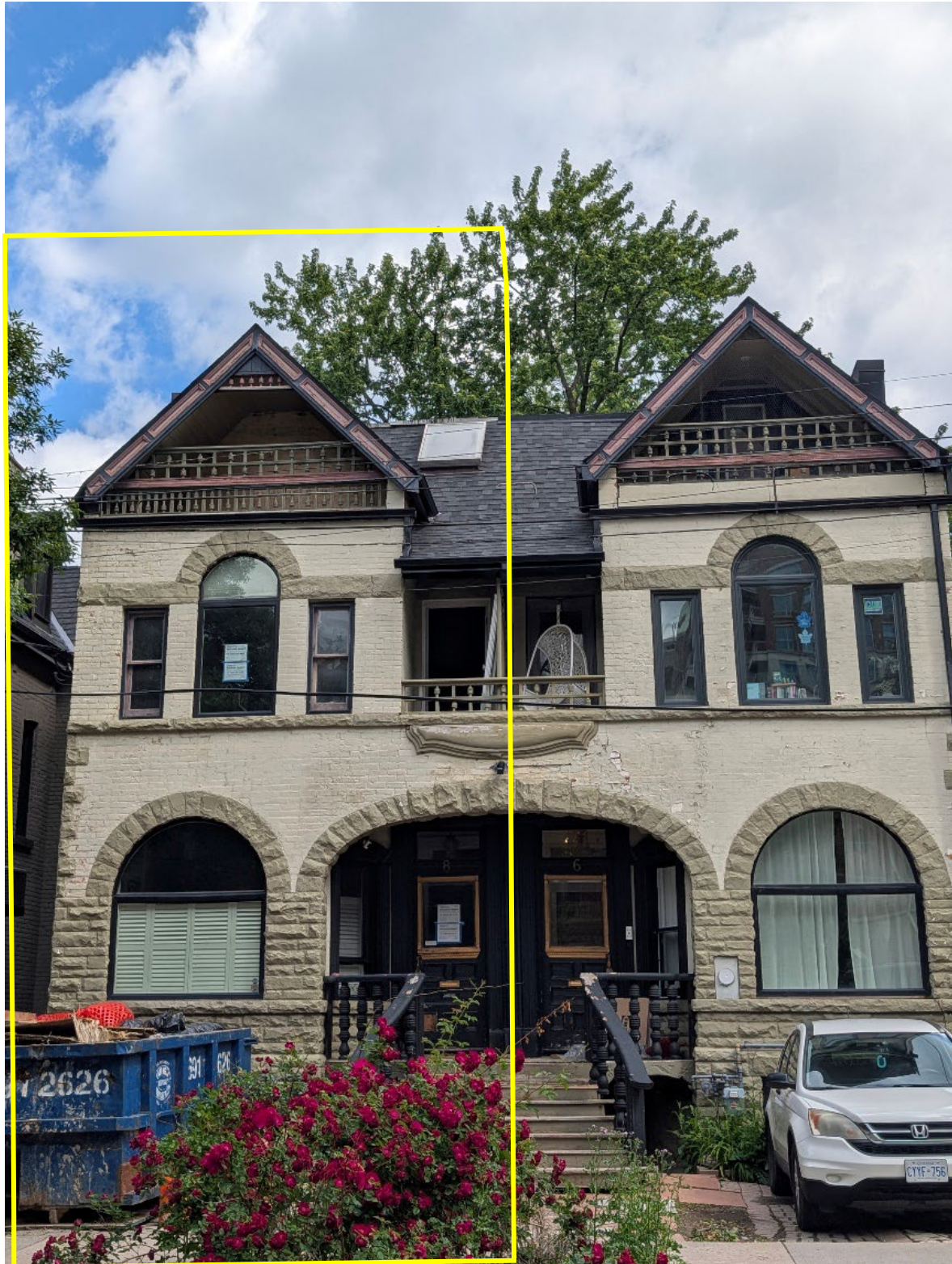
Primary (south) elevation of 8 Lowther Avenue outlined in yellow showing the building as seen from Lowther Avenue. (Heritage Planning, 2026)
