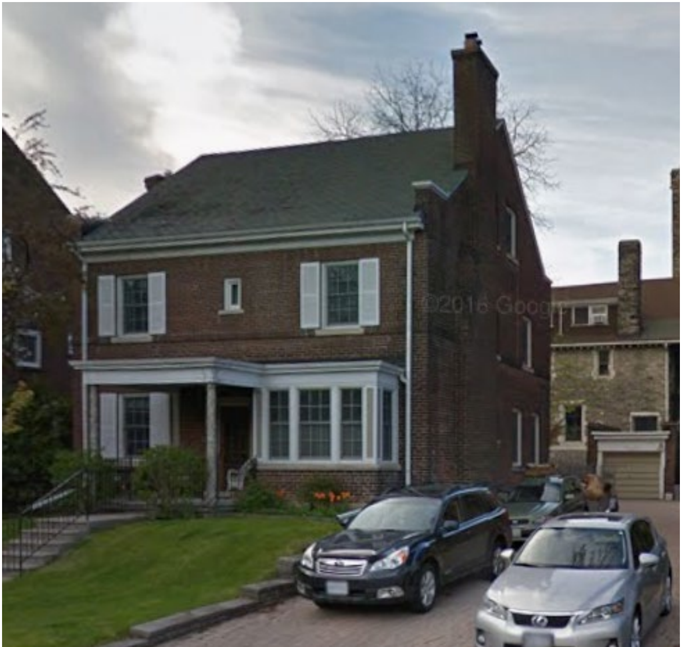
View of the principal elevation at 6 Whitney Avenue, showing preexisting garage at the rear (Google Maps, 2016).
