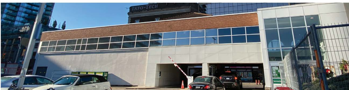
East (Rear) Elevation of the heritage façade (ERA Architects, 2021)
