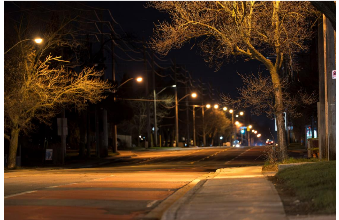
Conventional high-pressure sodium cobra head: Kennedy Road (between Eglinton & Lawrence)
