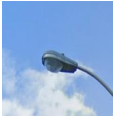
Conventional cobra head (high-pressure sodium) luminaires are the predominant fixture in the horseshoe
