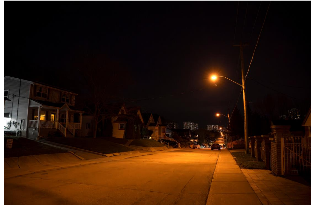
Conventional high-pressure sodium cobra head: Pitt Avenue
