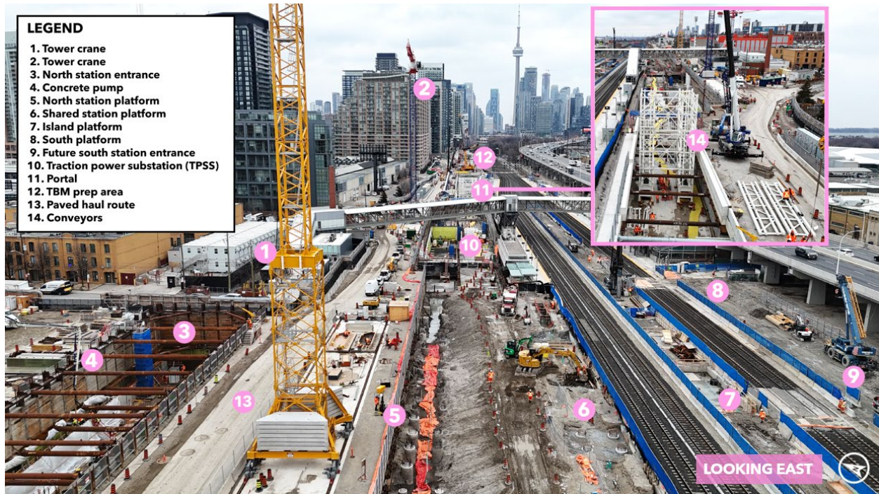
Figure 1: Current view looking east across Exhibition Station and portal works
