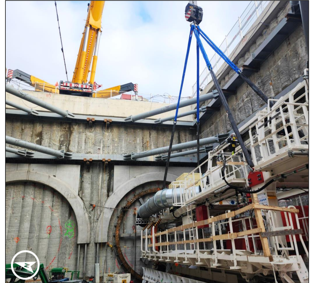
A view of the TBM gantry lift into the portal.
