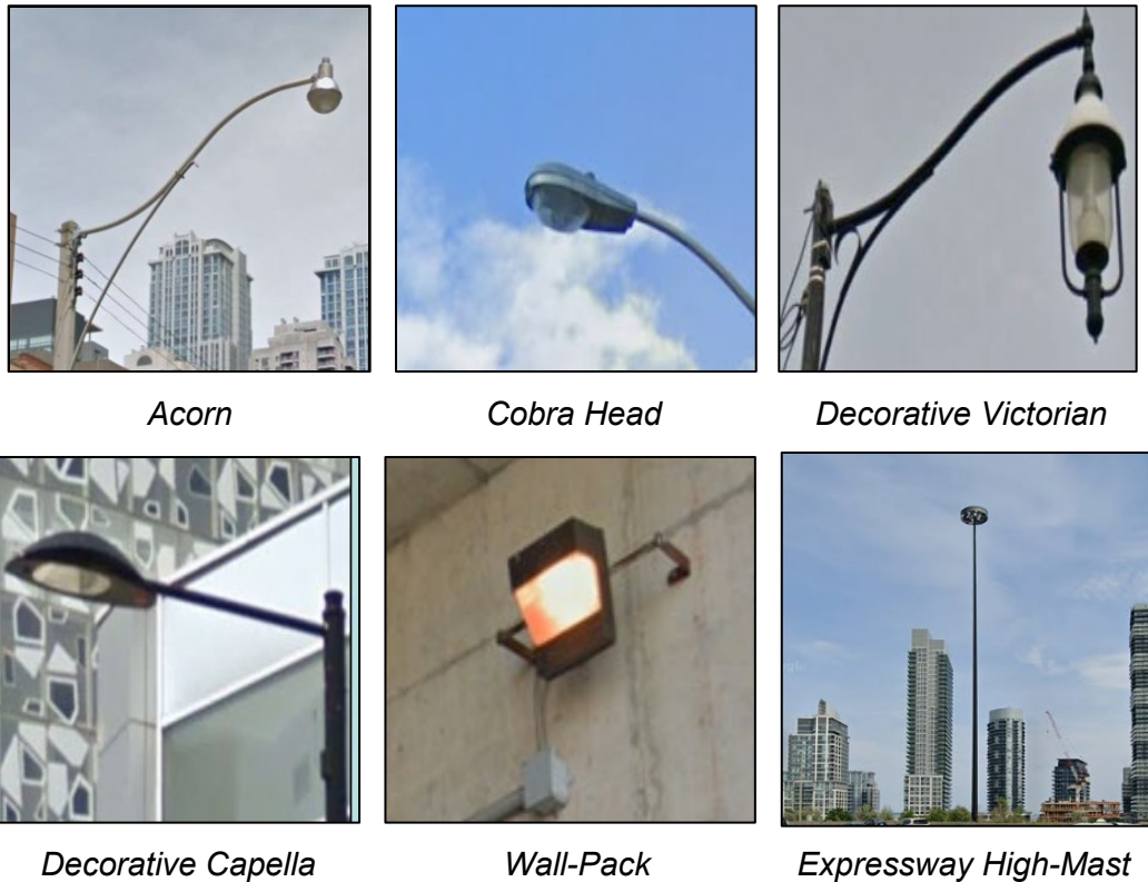
Figure 9: Typical Luminaire Types
