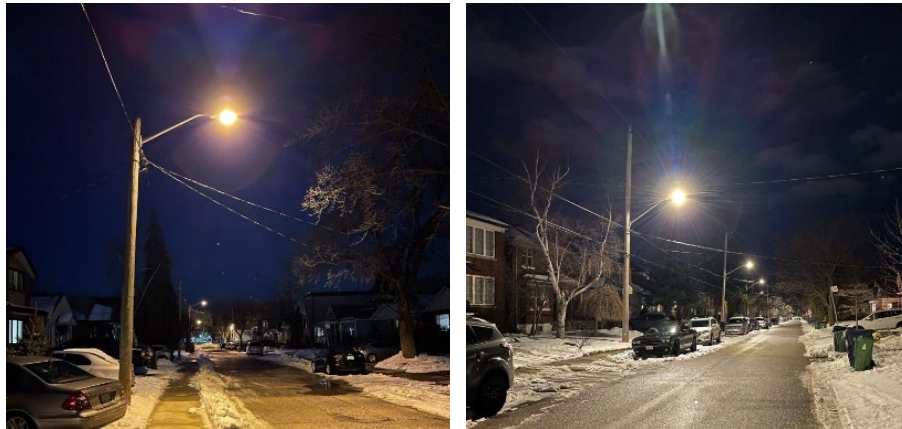
City of Toronto - Lakeshore & Islington Area Before (left) and After (right) LED Conversion.
