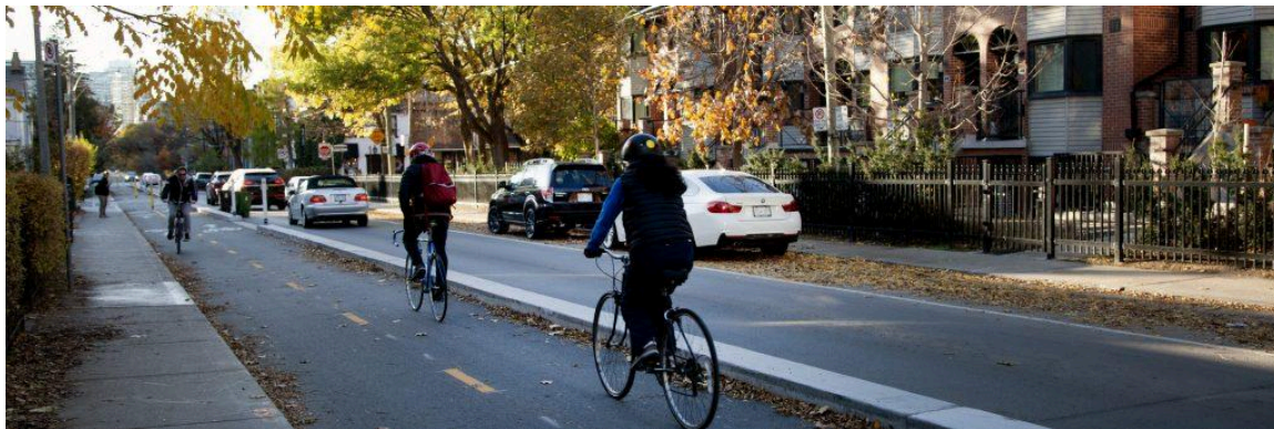
(Wellington protected bike lanes with poured concrete. Image: City of Toronto)
