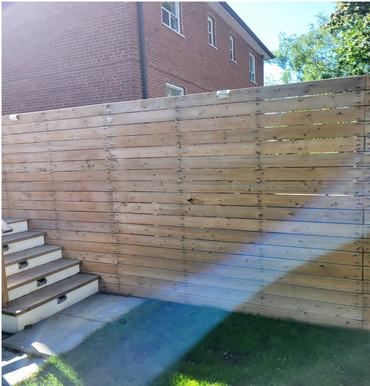
Attachment 4: South side fence adjacent to steps leading to deck rear yard. Photo taken by officer. 22 Ninth Street, City of Toronto.
