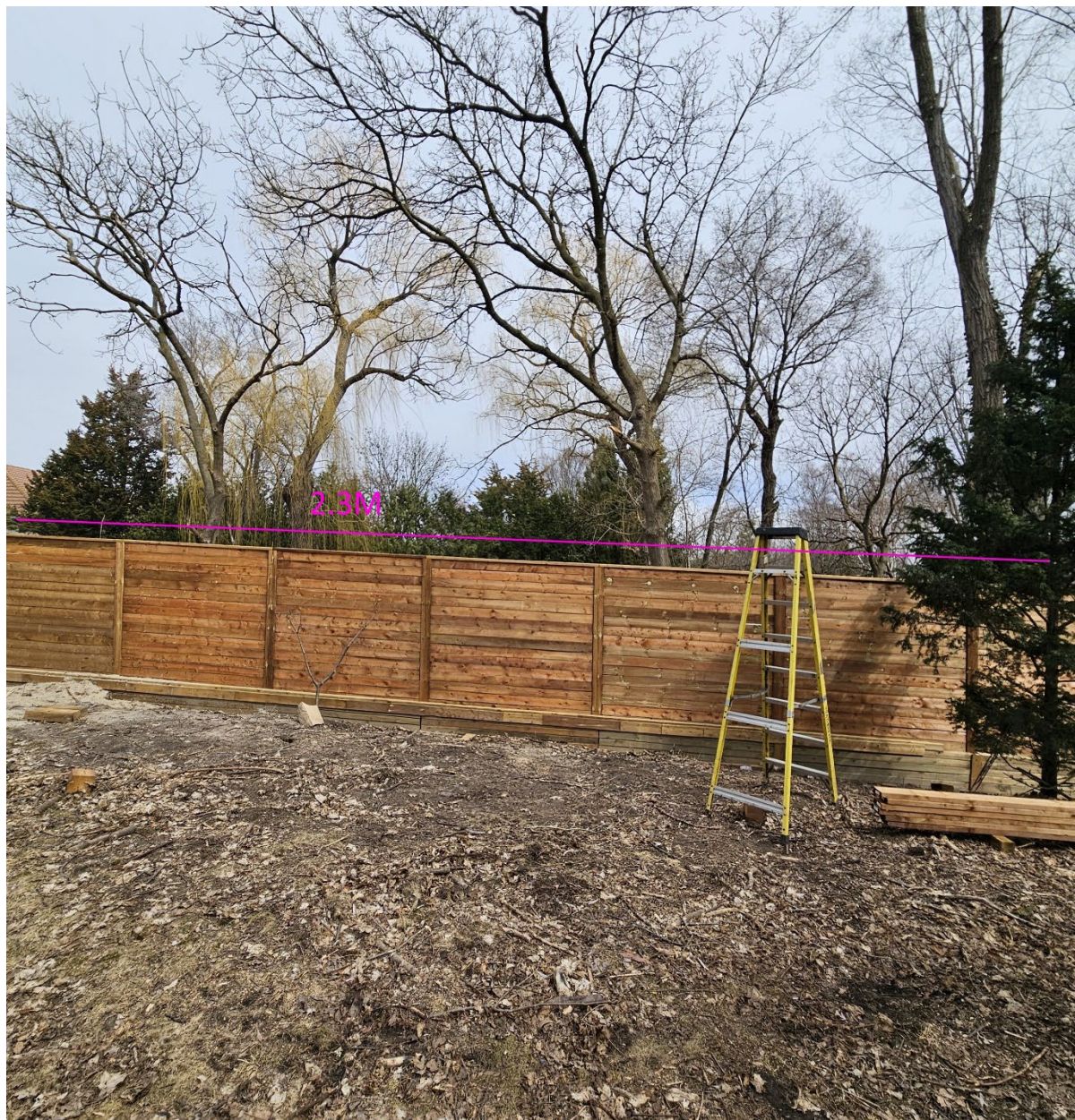
Attachment 3: Northeast rear yard. Photo taken by officer. 5 Alderton Court, City of Toronto.
