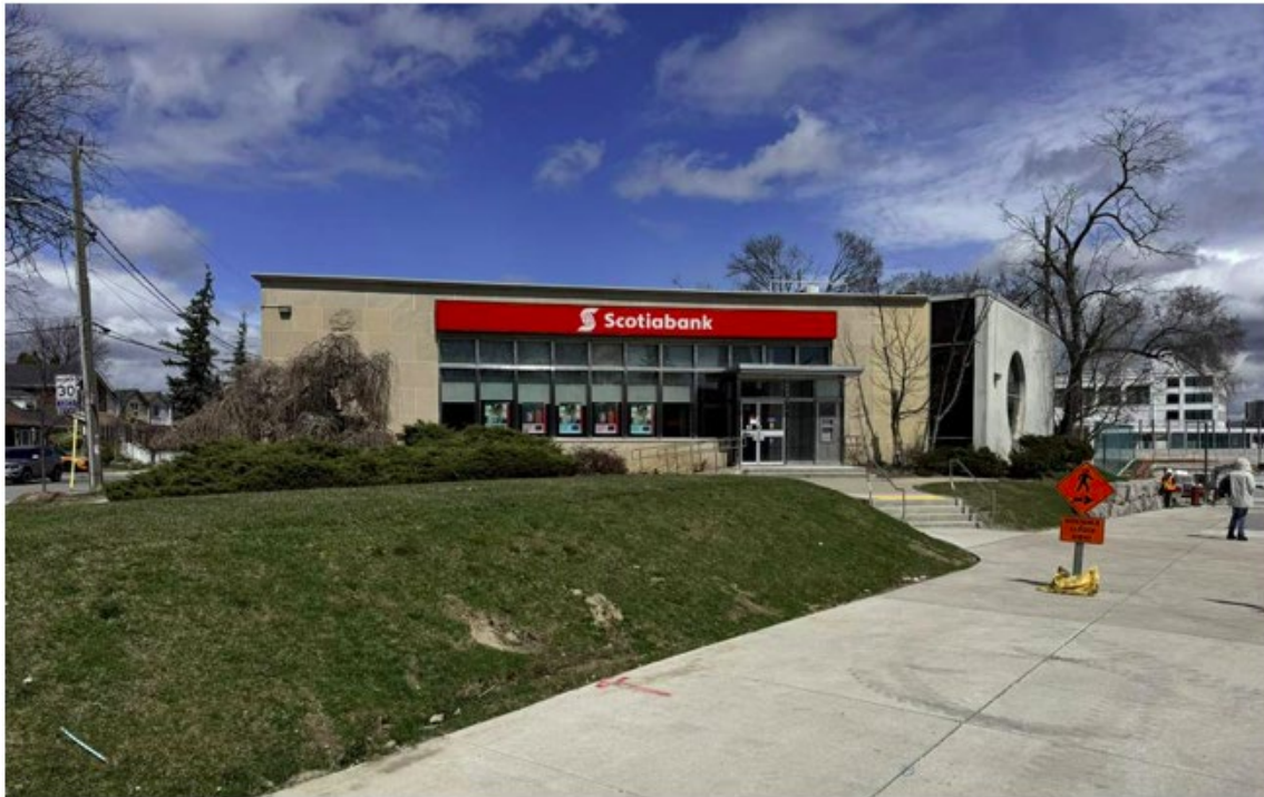
Primary elevation of 1151 Weston Road. The 1980s north wing is shown on the left side (HIA by Giaimo, March 2026).
