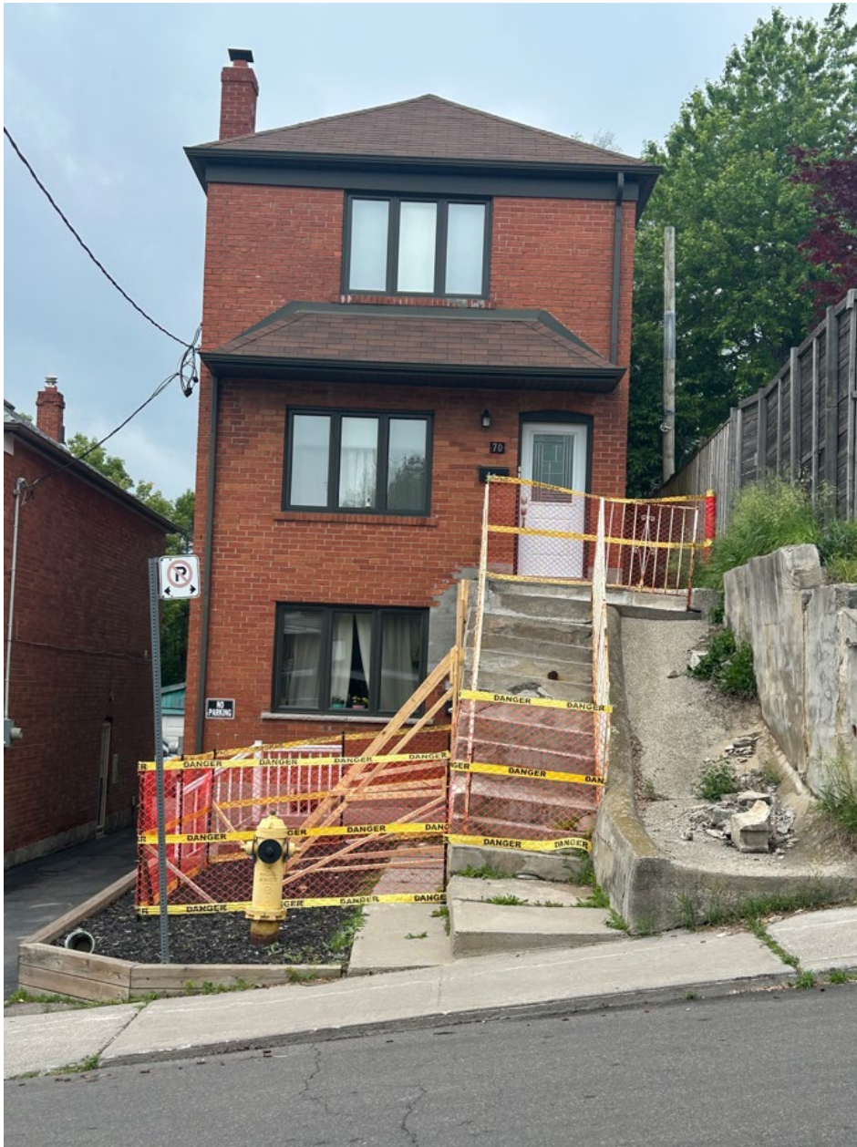
Looking west at 70 Lacey Avenue.
