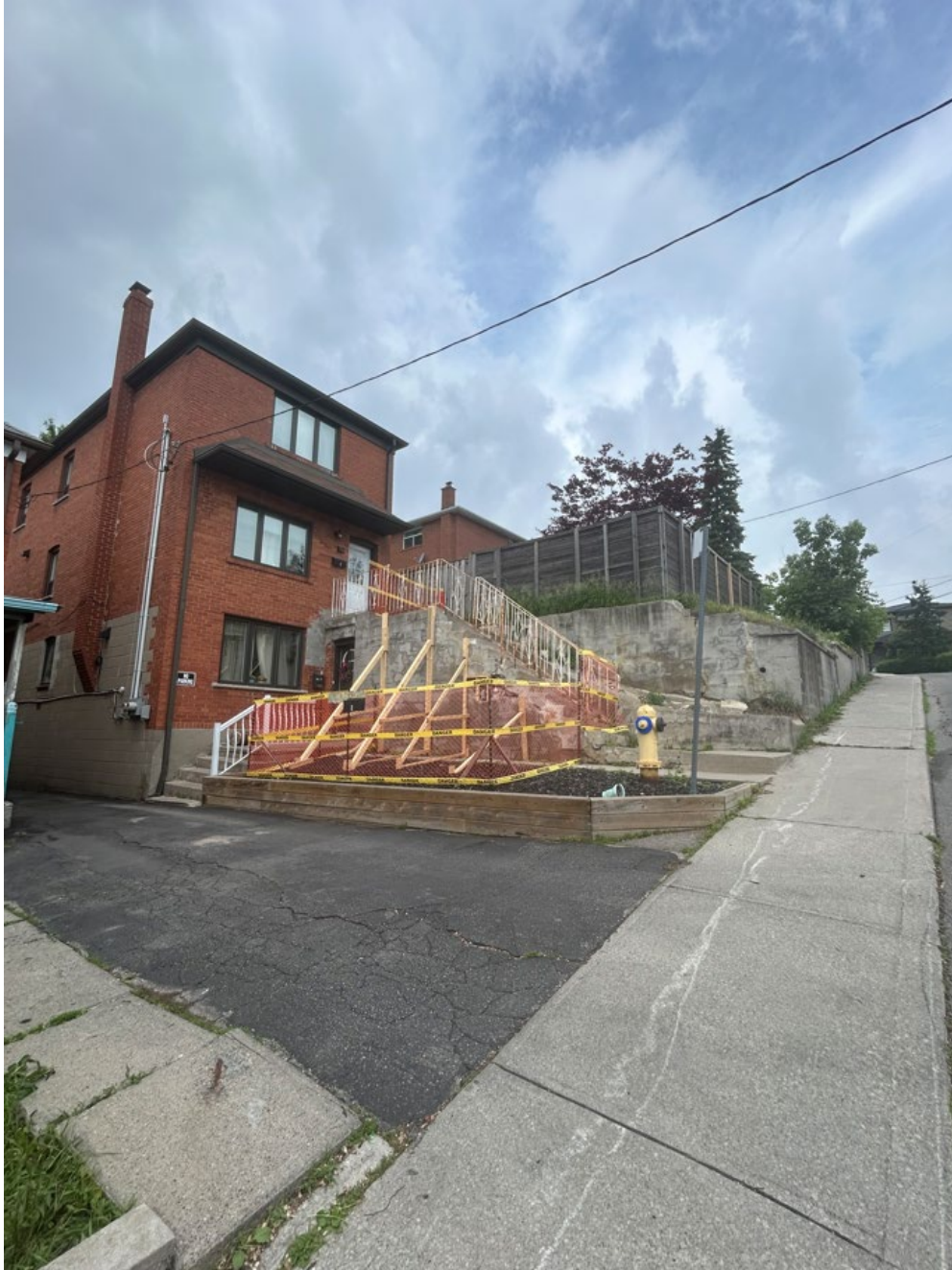
Looking North at 70 Lacey Avenue.
