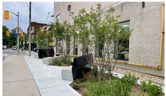
Precedent: Bloor West Village Parkette at Armadale Ave is developed in collaboration with Bloor West Village BIA. It features seating and tree planting, providing relief along the busy main street. (Credit: City of Toronto)
