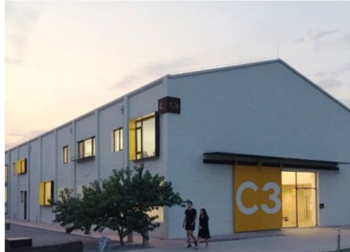
Figure 2.18: Beijing Enlight Media Workshop C3, Beijing, China.
