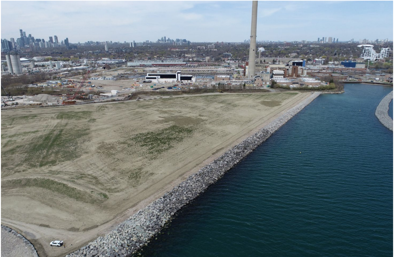
Figure 3 – Newly constructed Landform at the Ashbridges Bay Treatment Plant.
