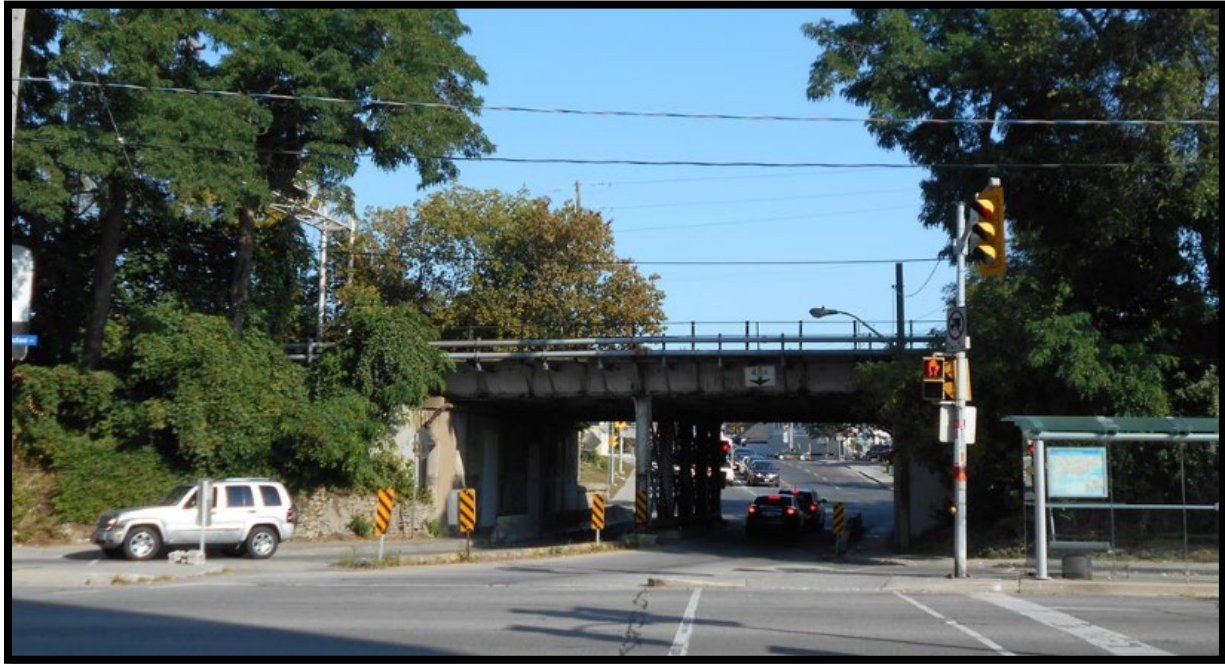
Figure 2: Scarlett Road Underpass, Elevation Photo Looking North along Scarlett Road from Dundas Street
