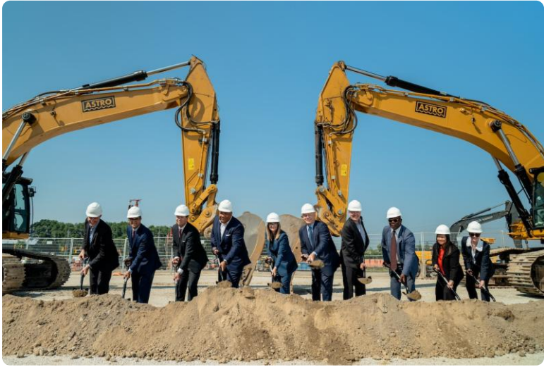
Alta at Scarborough Town Centre
