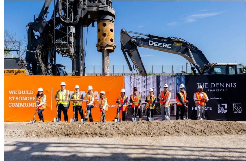
2025 groundbreaking on over 400 homes at 8-16 Locust St., in York-South Weston
