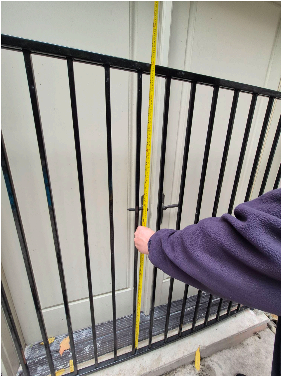
Attachment 9: Supervisor's photo – Rear Yard – Juliette style guard (2) height (1.5 meters)
