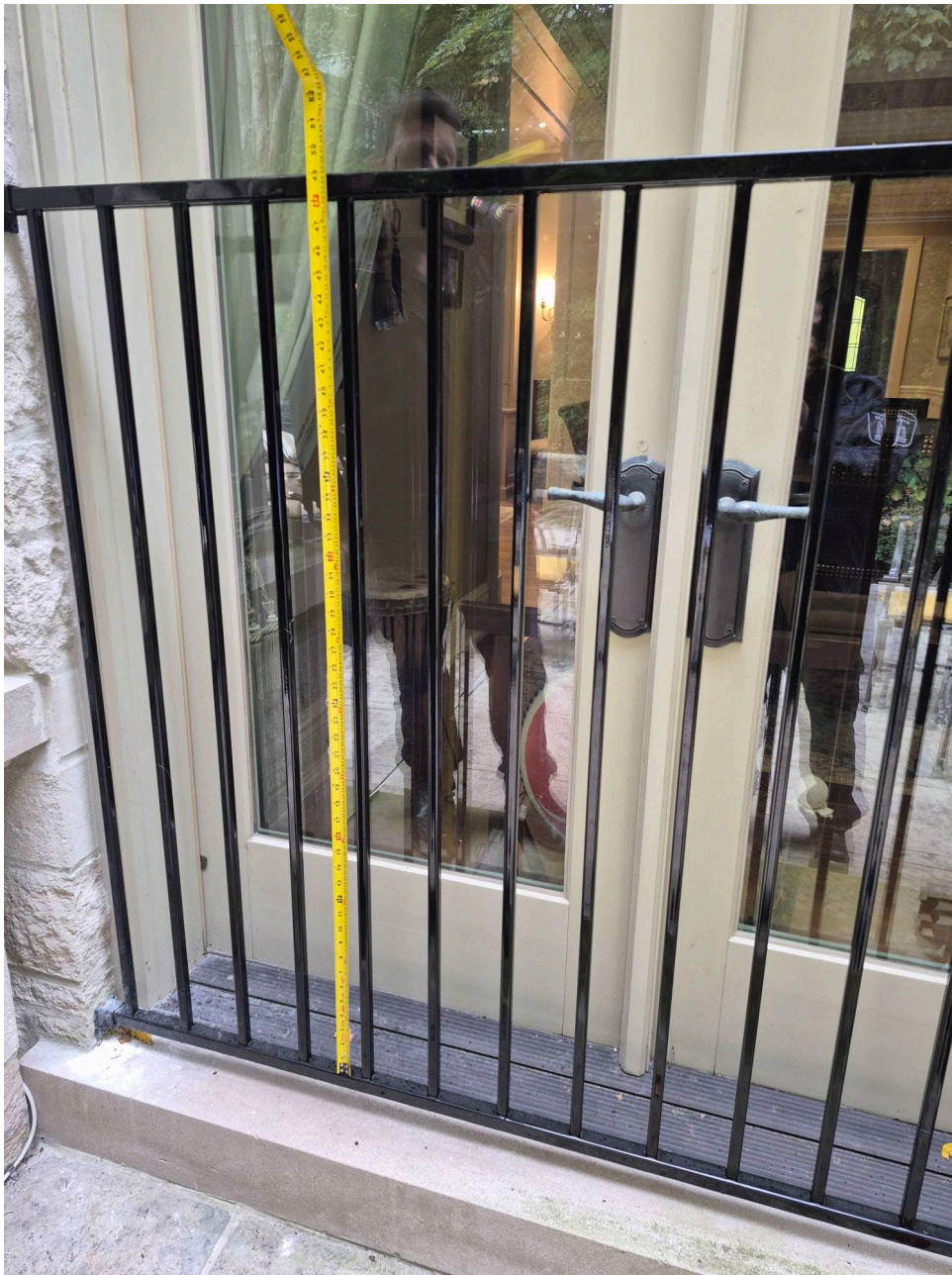
Attachment 7: Supervisor's photo – Rear Yard – Juliette style guard (1) height (1.25 meters)
