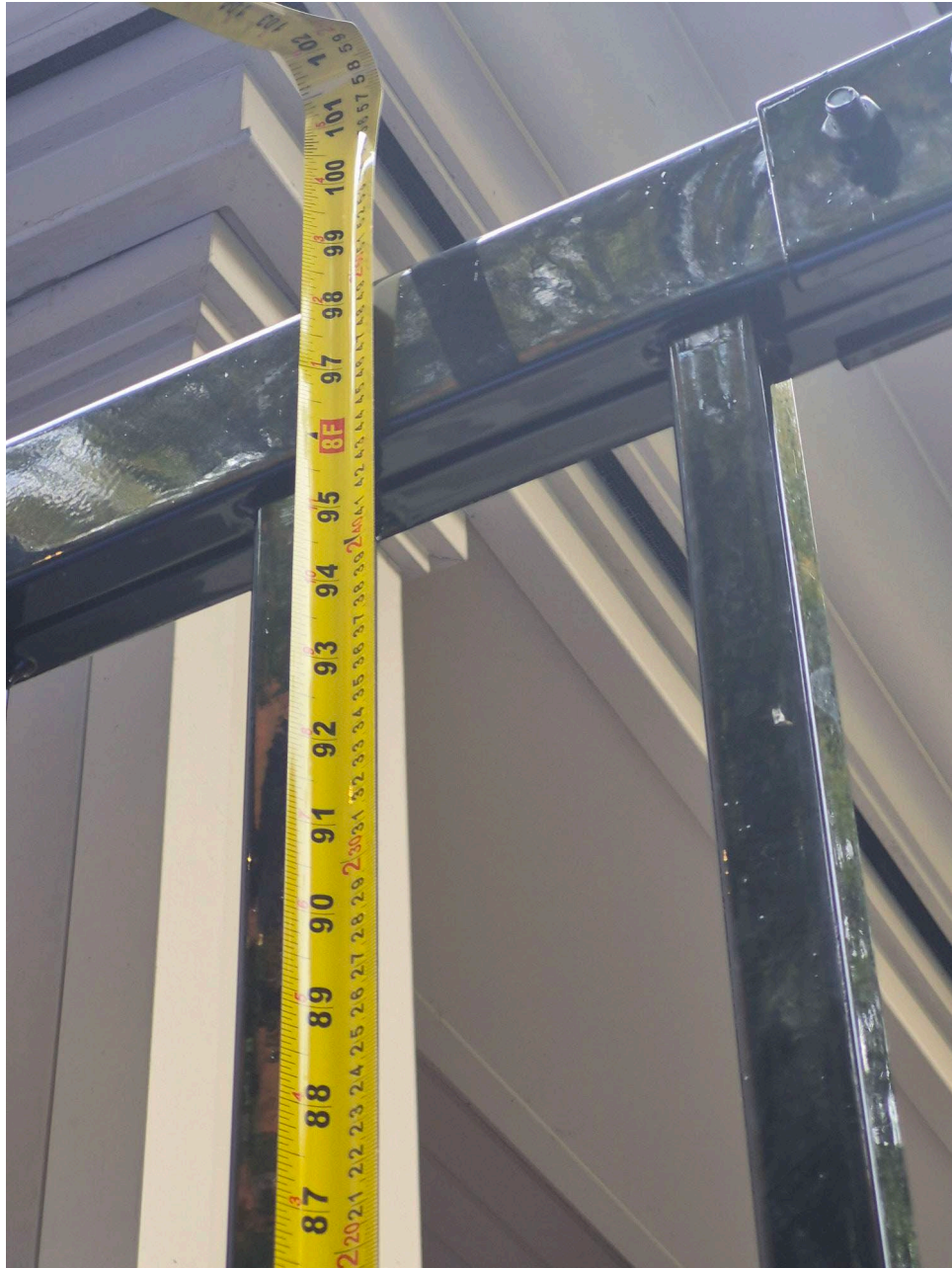
Attachment 5: Supervisor's photo – North side yard fence height. (2.49 meters)
