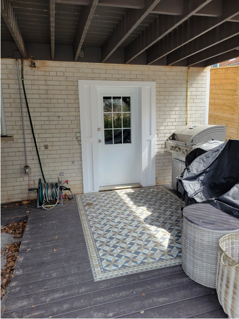
Attachment D: Rear west facing egress from property. Proposed gate location. Taken by Municipal Licensing and Standard Staff.
