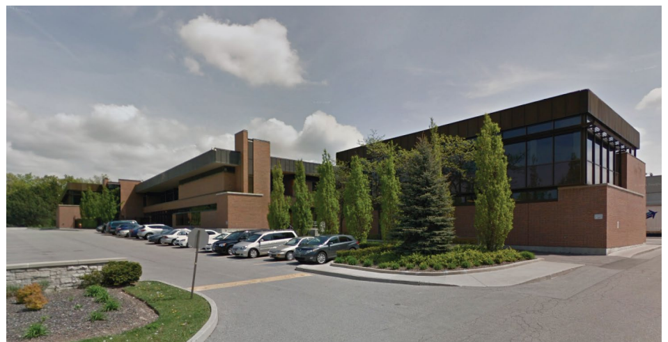
1123 Leslie Street Office Building
