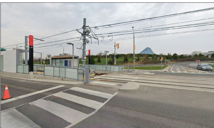
Eglinton Avenue East, looking north, Aga Khan Park & Museum Stop
