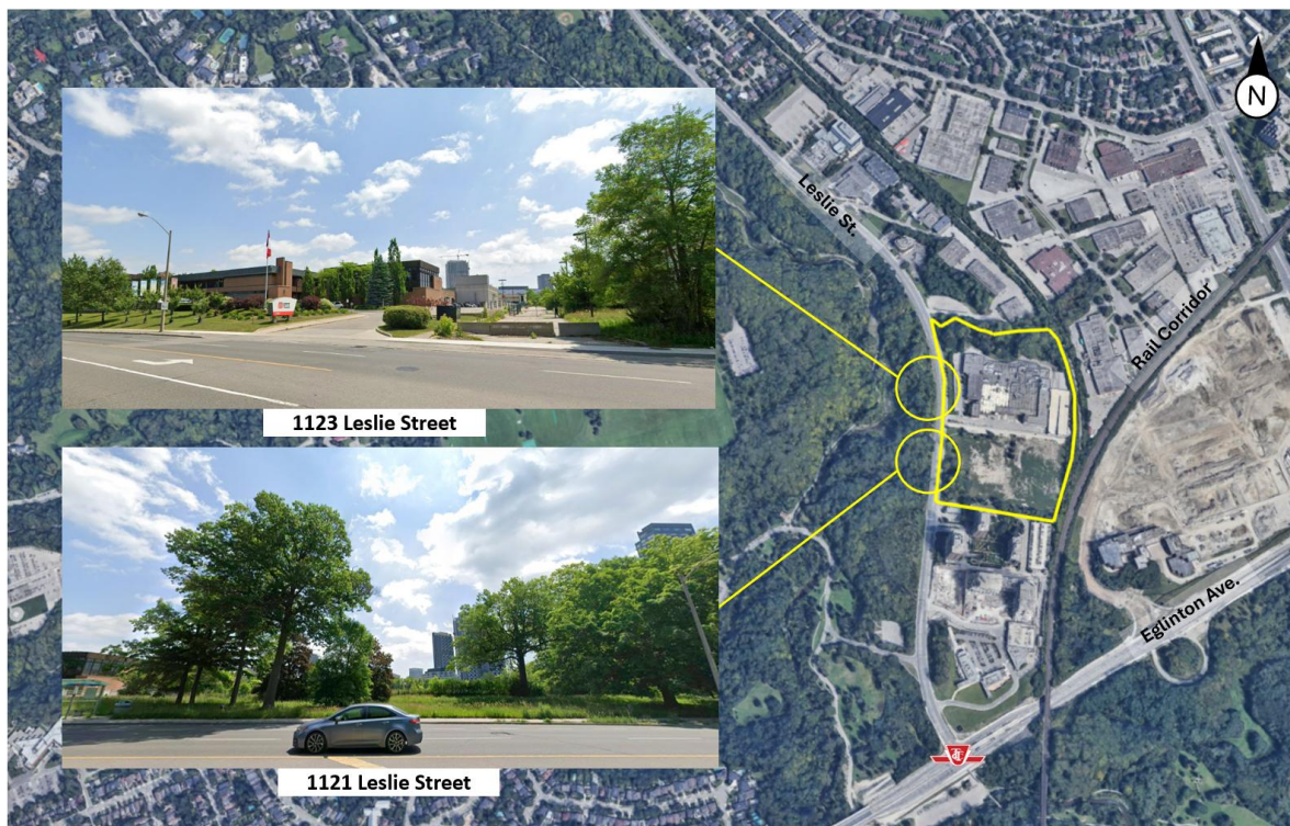
Figure 6: Street View of Leslie Site Properties
