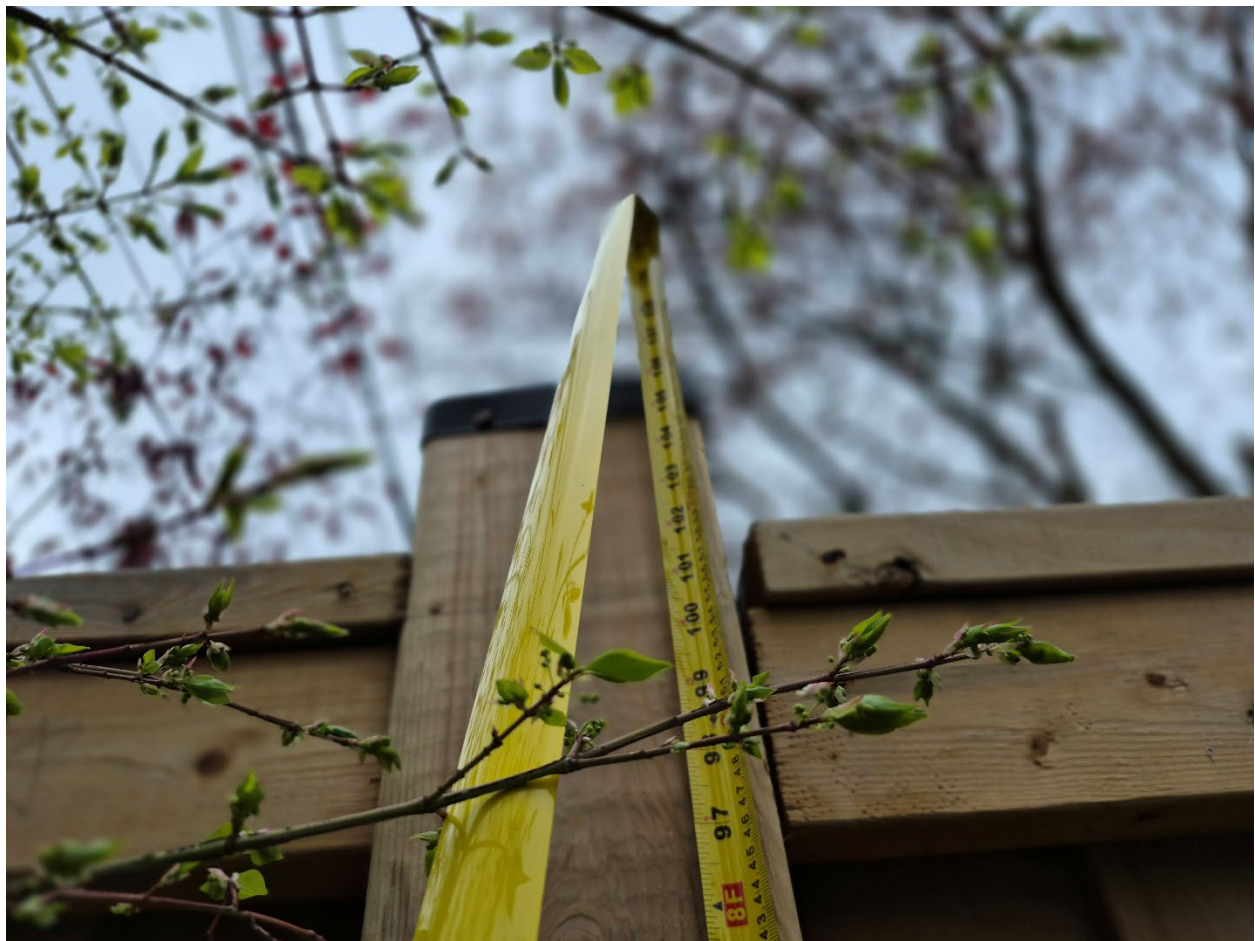
Attachment 5: Supervisor's photo - Rear yard fence- south side - fence height (2.51 meters to 2.69 meters)
