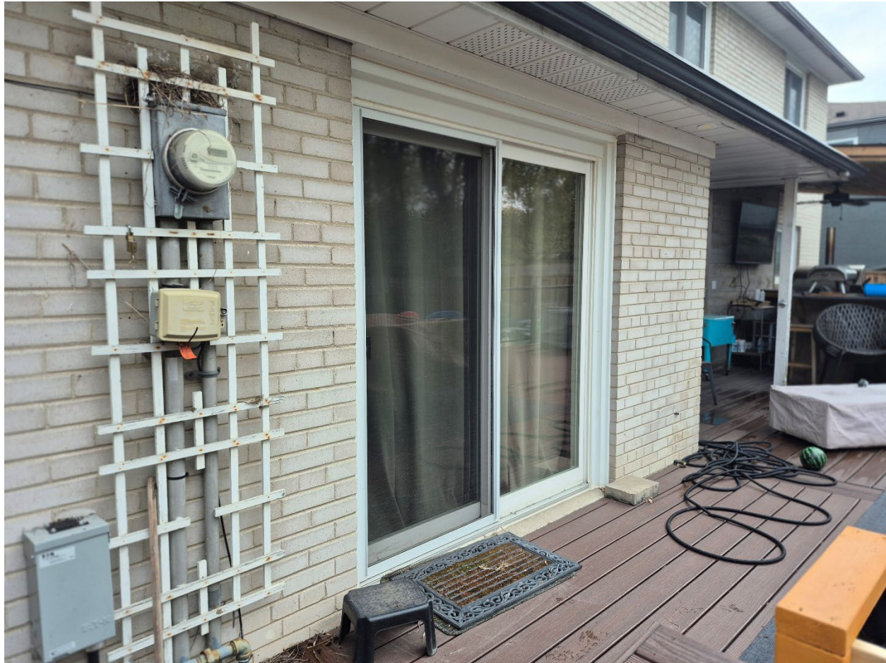
Attachment 6: Supervisor's photo - Overview of rear yard sliding door- North side
