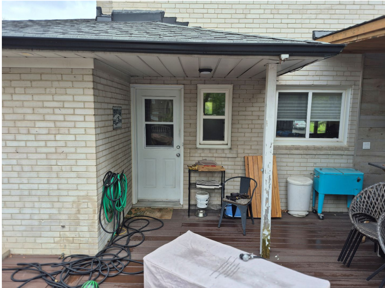
Attachment 8: Supervisor's photo - Overview of rear yard main door- North side
