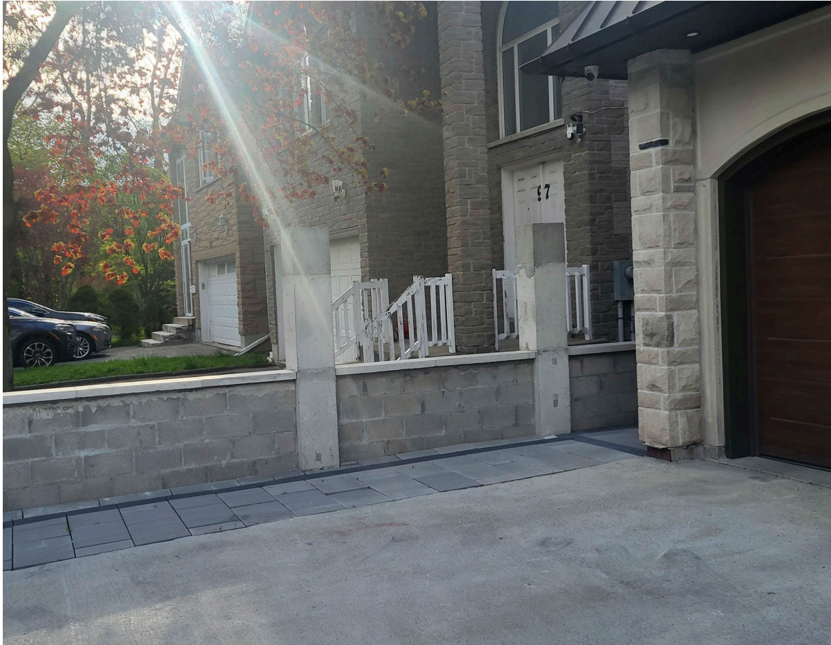
Attachment 7: East view of concrete cinder blocks and pillars. Photograph taken by Officer -101 Drewry Avenue - City of Toronto.
