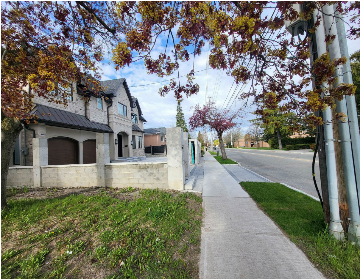
Attachment 2: East full view of the sidewalk showing the concrete cinder block wall and pillars. Photograph taken by Officer - 101 Drewry Avenue - City of Toronto.
