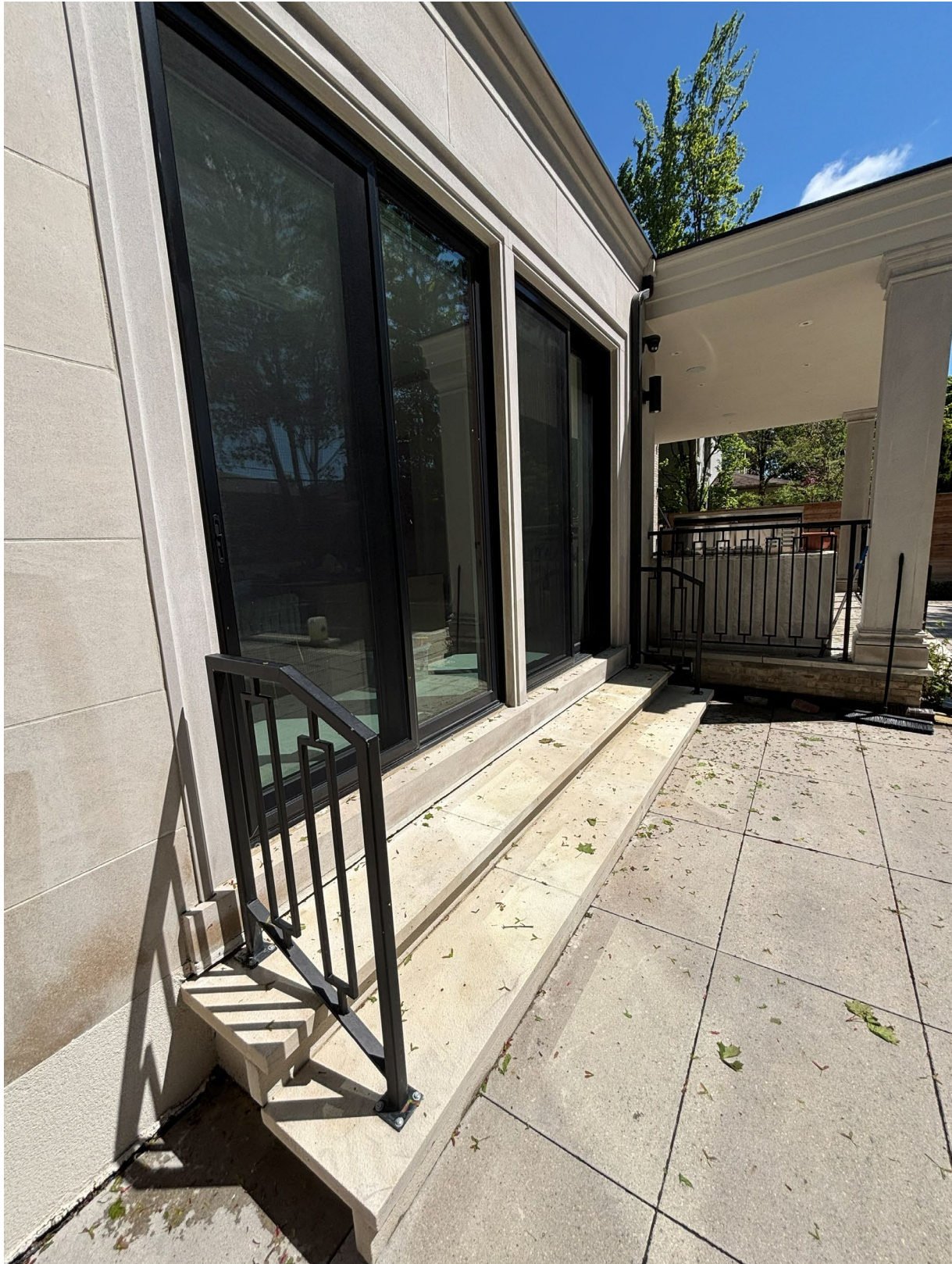
Attachment 8: South facing walkout access point without gate – 2 sliding doors.
