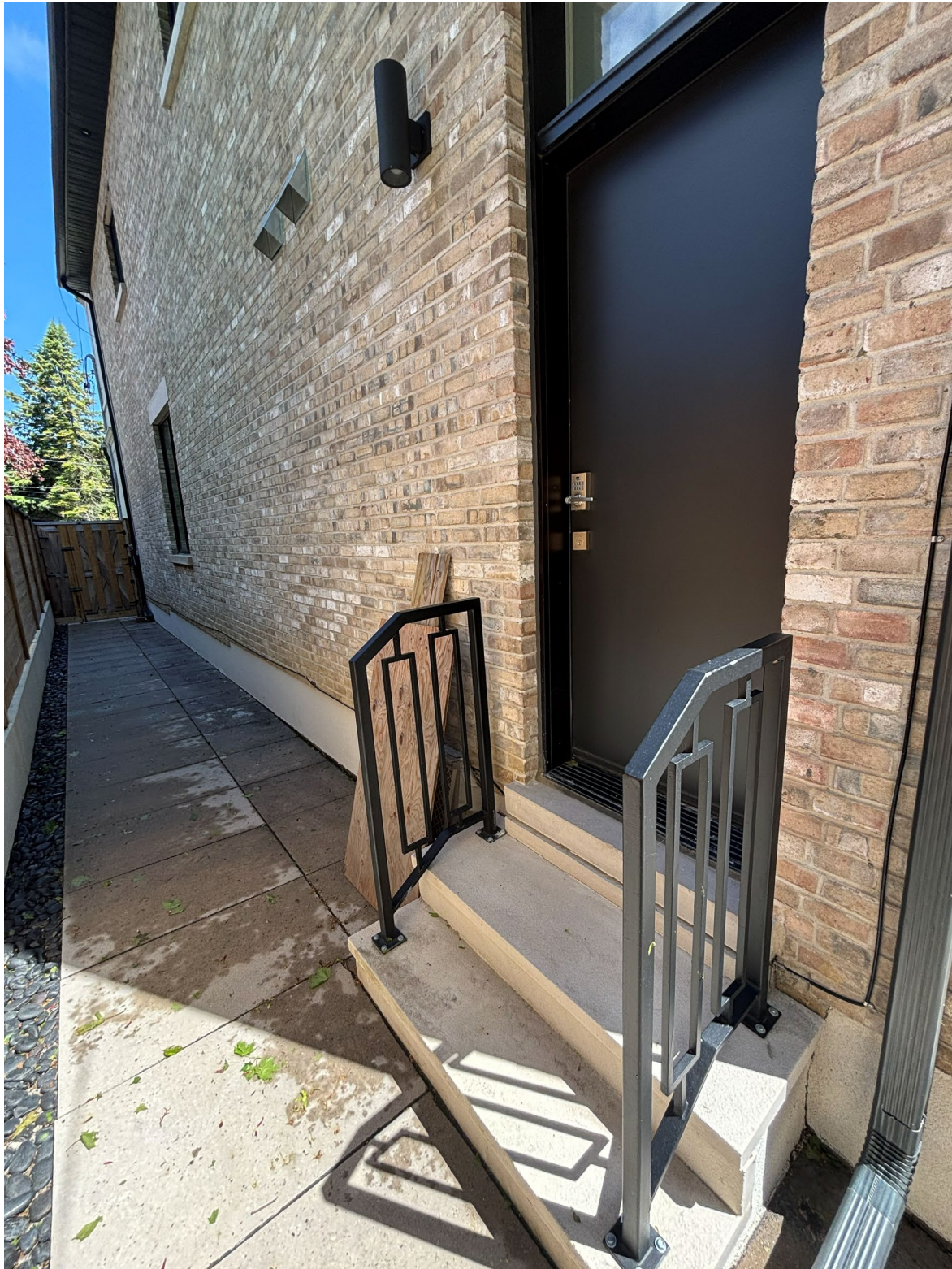
Attachment 7: West facing side walkout access point without gate (south-west corner of building).
