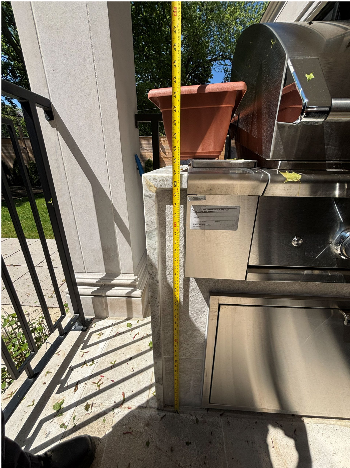
Attachment 10: Exterior BBQ and counter less than 1 meter away from forth fence.
