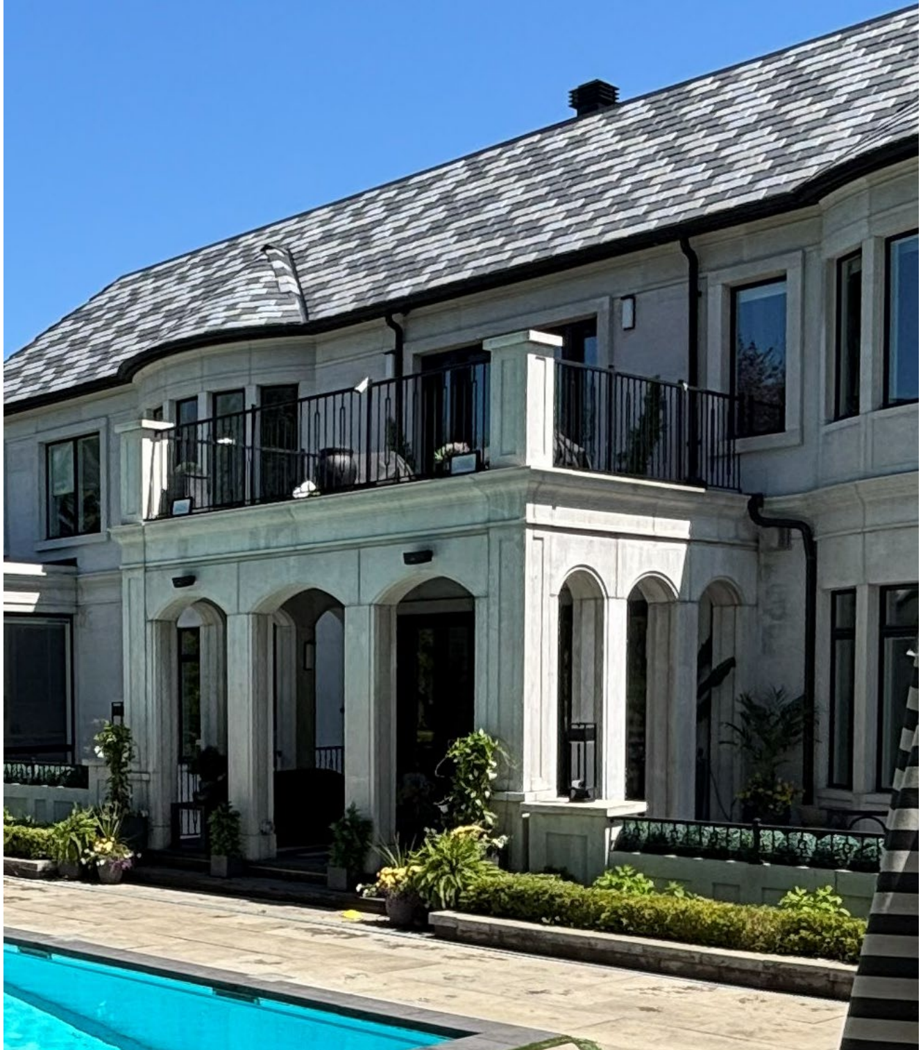
Attachment 4: Rear yard covered patio - west facing sliding doors from ground/main level with six (6) column openings without any pool fence enclosure.
