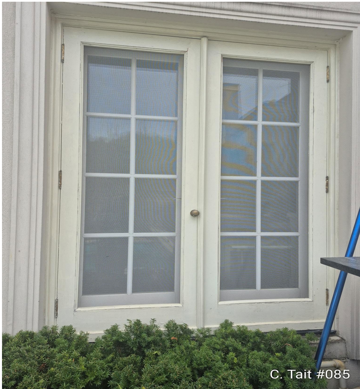
Attachment F: Door from dwelling into pool area. Taken by Municipal Standards staff.
