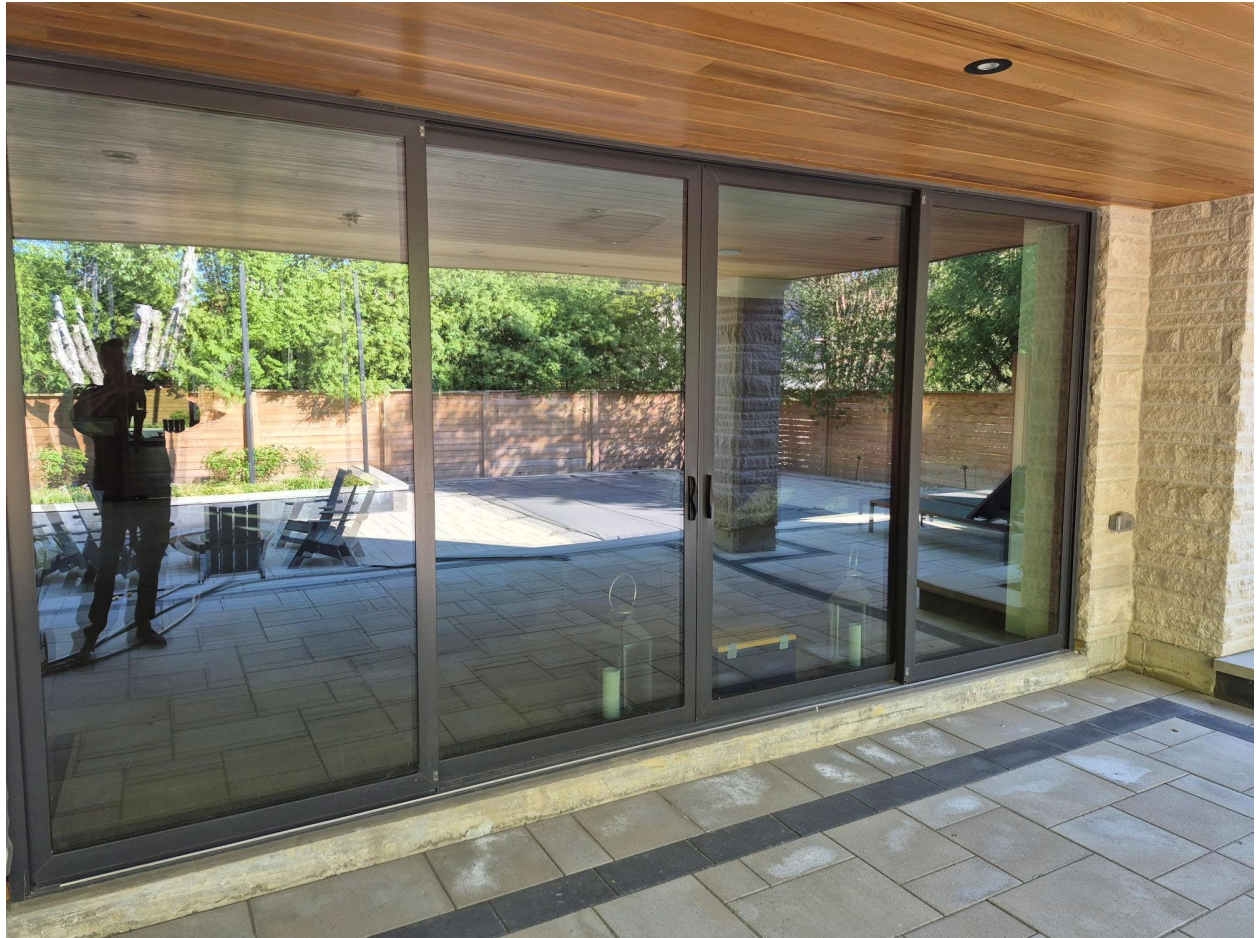
Attachment 6: Supervisor's photo - Overview of rear yard sliding door- Basement
