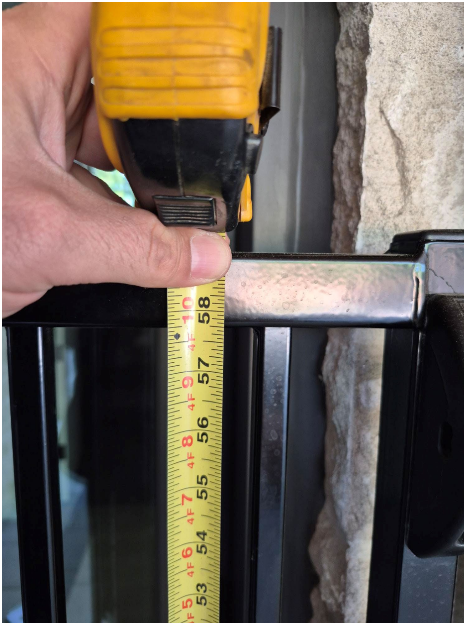
Attachment 8: Supervisor Photo - Rear yard door with Juliette style gate- Basement - Height (1.47 meters)
