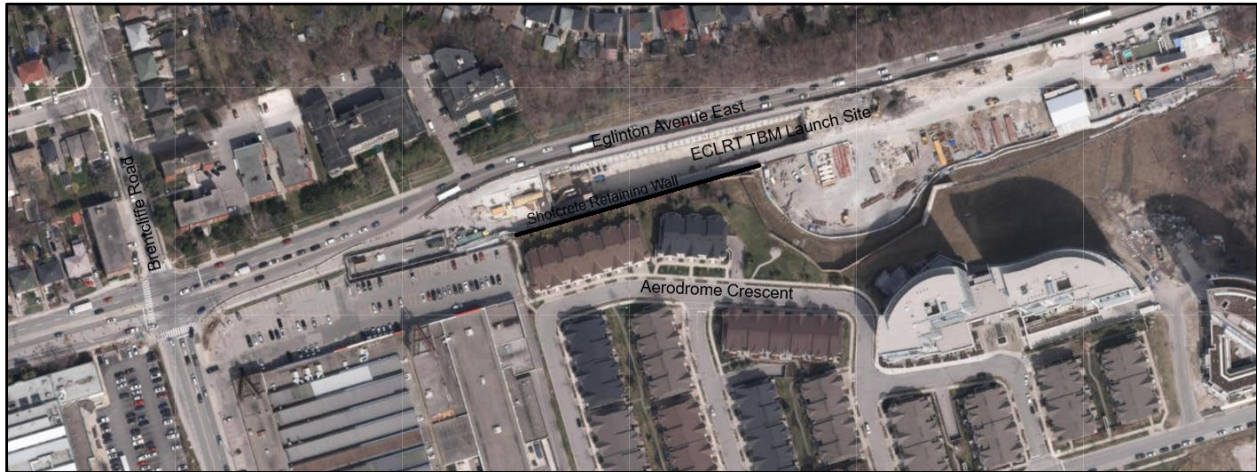
Figure 1 – Brentcliffe Shotcrete Wall during ECLRT Construction
