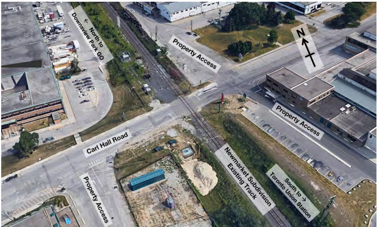
Figure 3 Existing Carl Hall Road Rail Crossing
