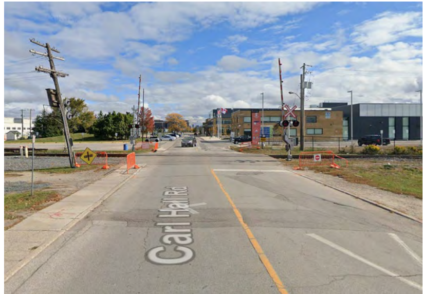
Existing Carl Hall Road at-grade rail crossing, looking east.
