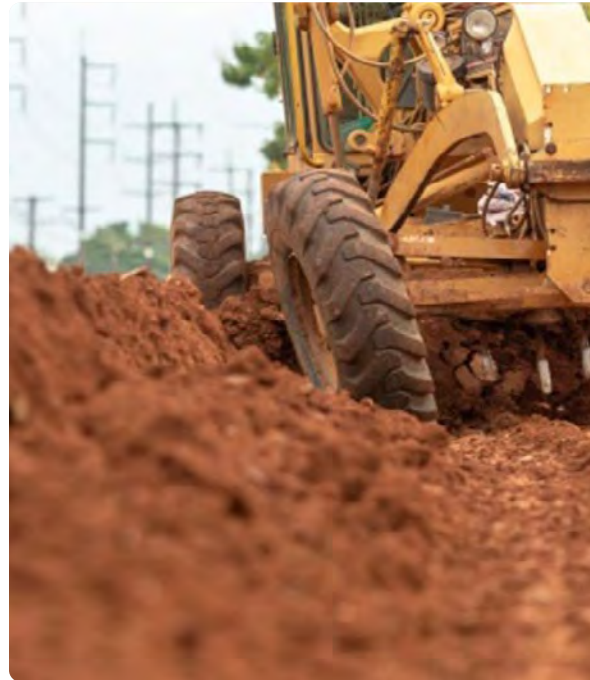
Figure 136: Re-grading soil within the site.
