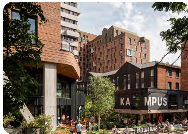
Figure 65: Industrial Character around the Depot, Manchester, England (ArchDaily).
