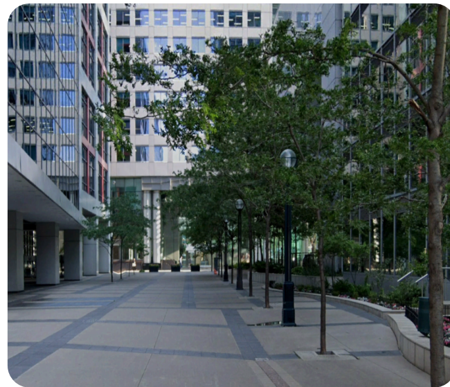
Figure 41: 200 Wellington Street, Toronto.
