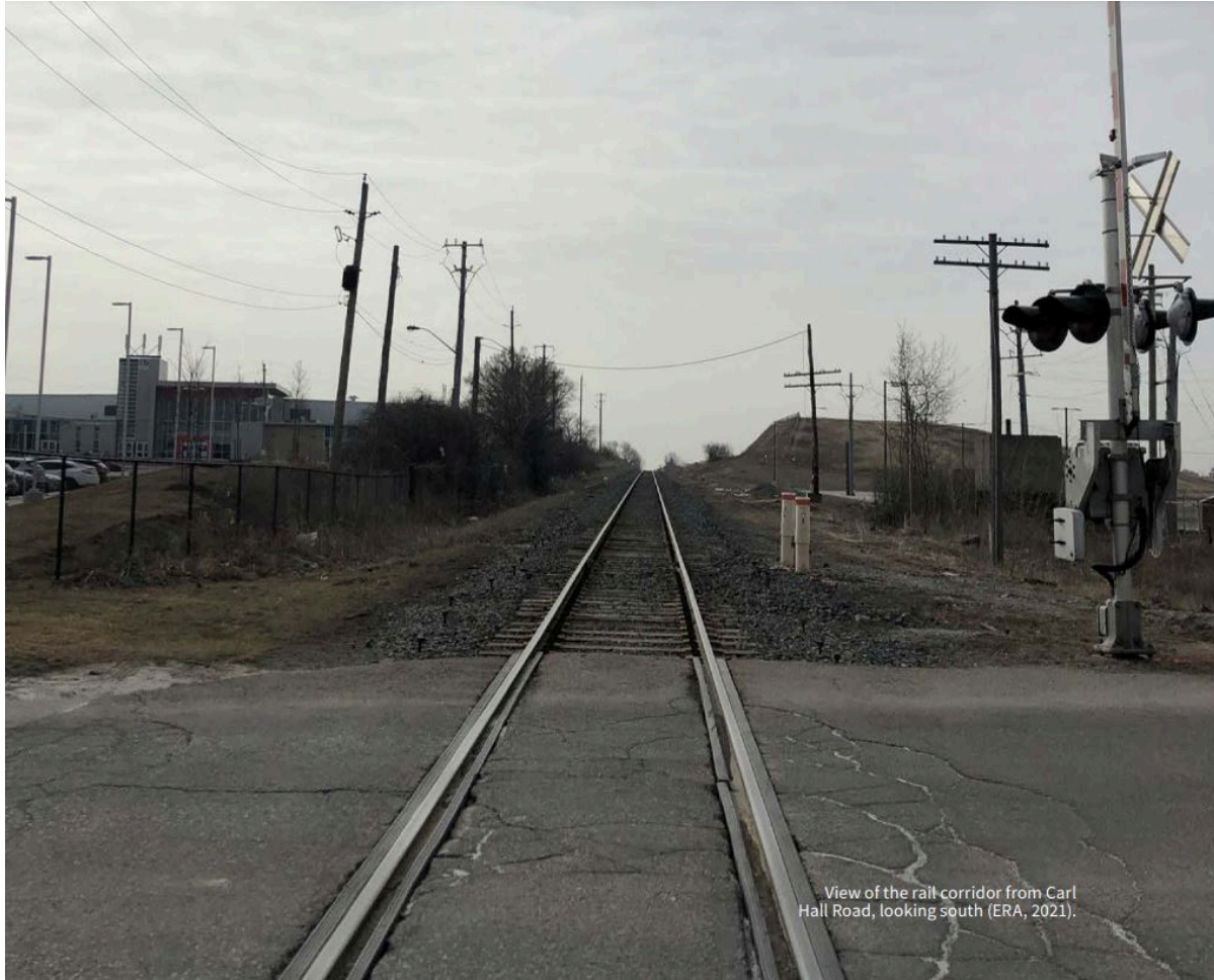
Figure 1: The Carl Hall Road crossing today “is an existing at-grade rail crossing and includes automatic warning devices such as Reflectorized Crossbucks (R), Flashing Lights (F), Bell (B), and Gates (G)”. (p12, Rail Safety and Risk Mitigation Report ).
