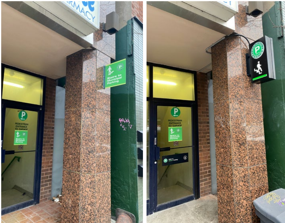
(Above – Figure 21) CP111 before and after with exterior signage for pedestrian entry/exit points that use new branding standards and graphic language with illuminated signage. (Right – Figure 22) CP34 before and after with exterior brand applications to better identify customer entry/exit points with new guideline sign elements. This eliminates confusion and identifies proper Green P car park sidewalk entries.
