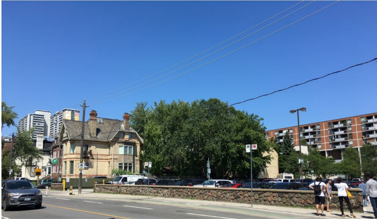
Figure 2. 405 Sherbourne Street looking northeast (ERA Architects Inc., 2020).
