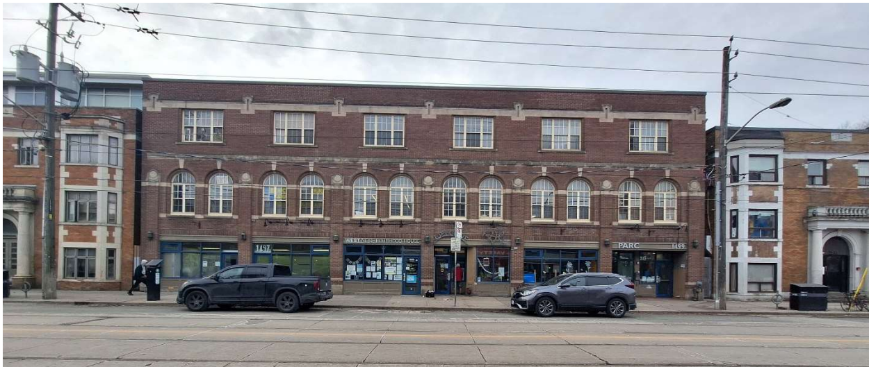
Figure 3 Principal (north) elevation of 1497 Queen Street West. Note the replacement windows at the second and third storeys match those in the 1924 and 1925 architectural drawings (Heritage Planning, 2025).
