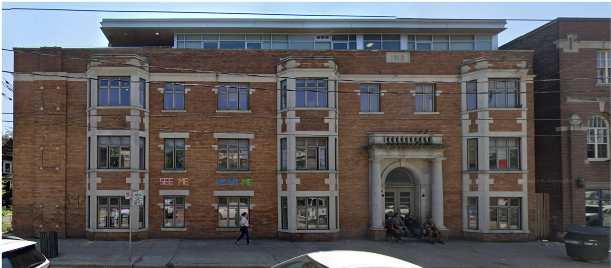
Figure 7 194 Dowling Avenue (Google Maps, 2023).
