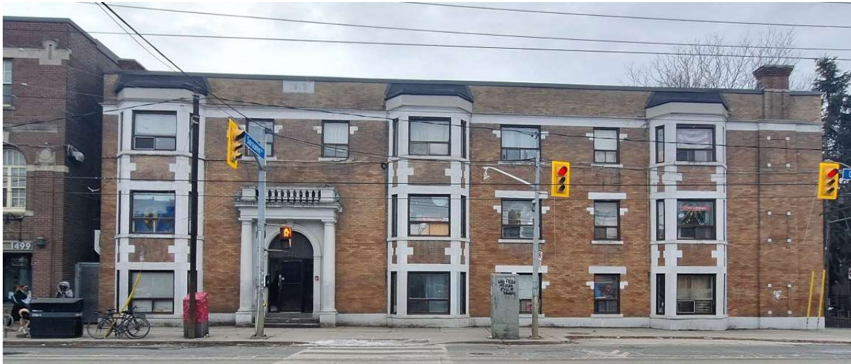
Figure 8 1501 Queen Street West (Heritage Planning, 2025).
