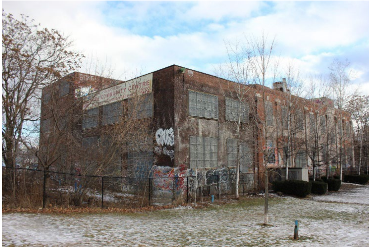
Figure 25. View of the northwest elevation looking southeast (Heritage Planning, 2025).
