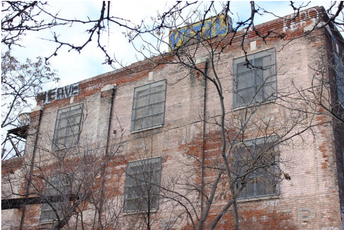
Figure 30. Detail of the south elevation of the Storage & Barrelling Refinery "ghost signage" lettering painted onto the bricks (Heritage Planning, 2025).
