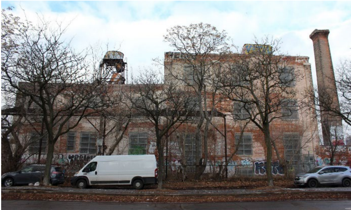
Figure 27. View of the south elevation looking north showing the two-storey Mill Building at left with the "lean-to" steel canopy frame structure below and grain hopper above, the three-storey Storage & Barrelling Refinery at right, and the Boiler House Chimney Stack at far right (Heritage Planning, 2025).
