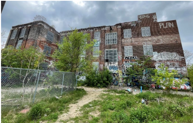
Figure 23. View of the east elevation showing the Storage & Barrelling Refinery, the Warehouse, and the c.1940 addition (Heritage Planning, 2024).
