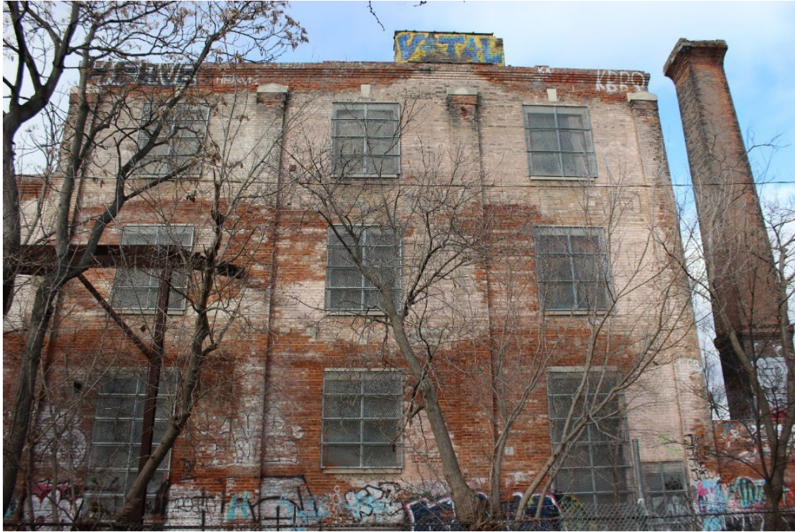
Figure 29. Detail view of the south elevation of the Storage & Barrelling Refinery showing the regular placement of the window openings and pilasters (Heritage Planning, 2025).
