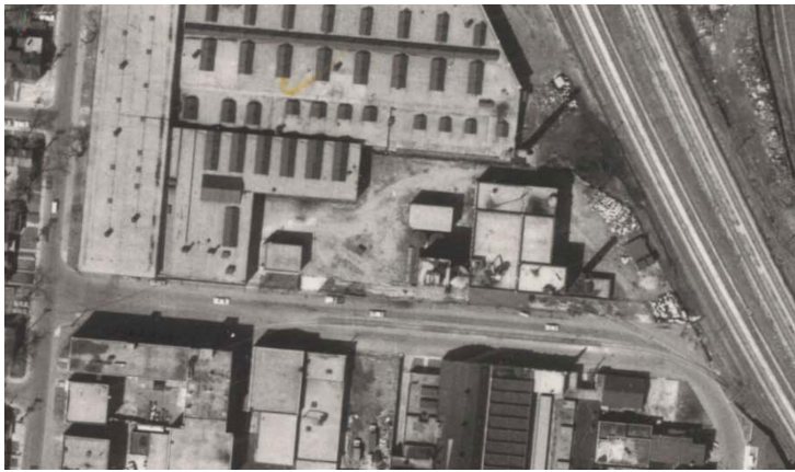
Figure 18. 1968 aerial photograph, plate 45, showing the property with the Tank House and Grain Elevator still intact (CTA).
