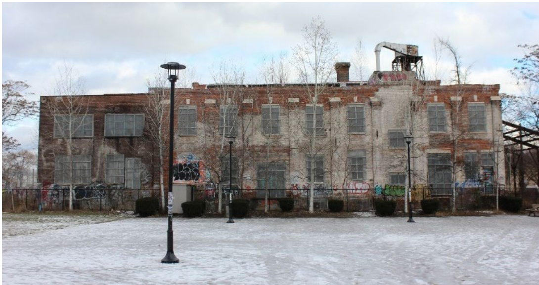
Figure 26. View of the west elevation looking east showing the different between the original c.1910 Mill building at right and the c.1941-47 rear addition at left (Heritage Planning, 2025).
