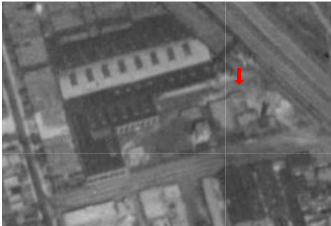
Figure 13. 1931 aerial of 40 Wabash Avenue showing the appearance of the Warehouse building (Toronto iView Mapping).
