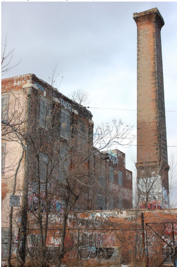
Figure 36. Detail view of the Boiler House Chimney Stack with corbelling details, its form and massing characteristic of the early 19th century industrial typology (Heritage Planning, 2025).
