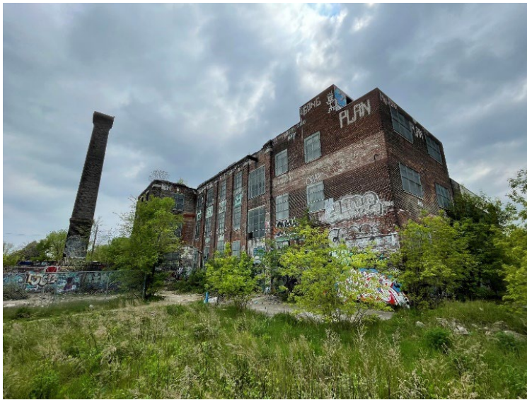
Figure 24. View of the northeast elevation looking southwest (Heritage Planning, 2024).
