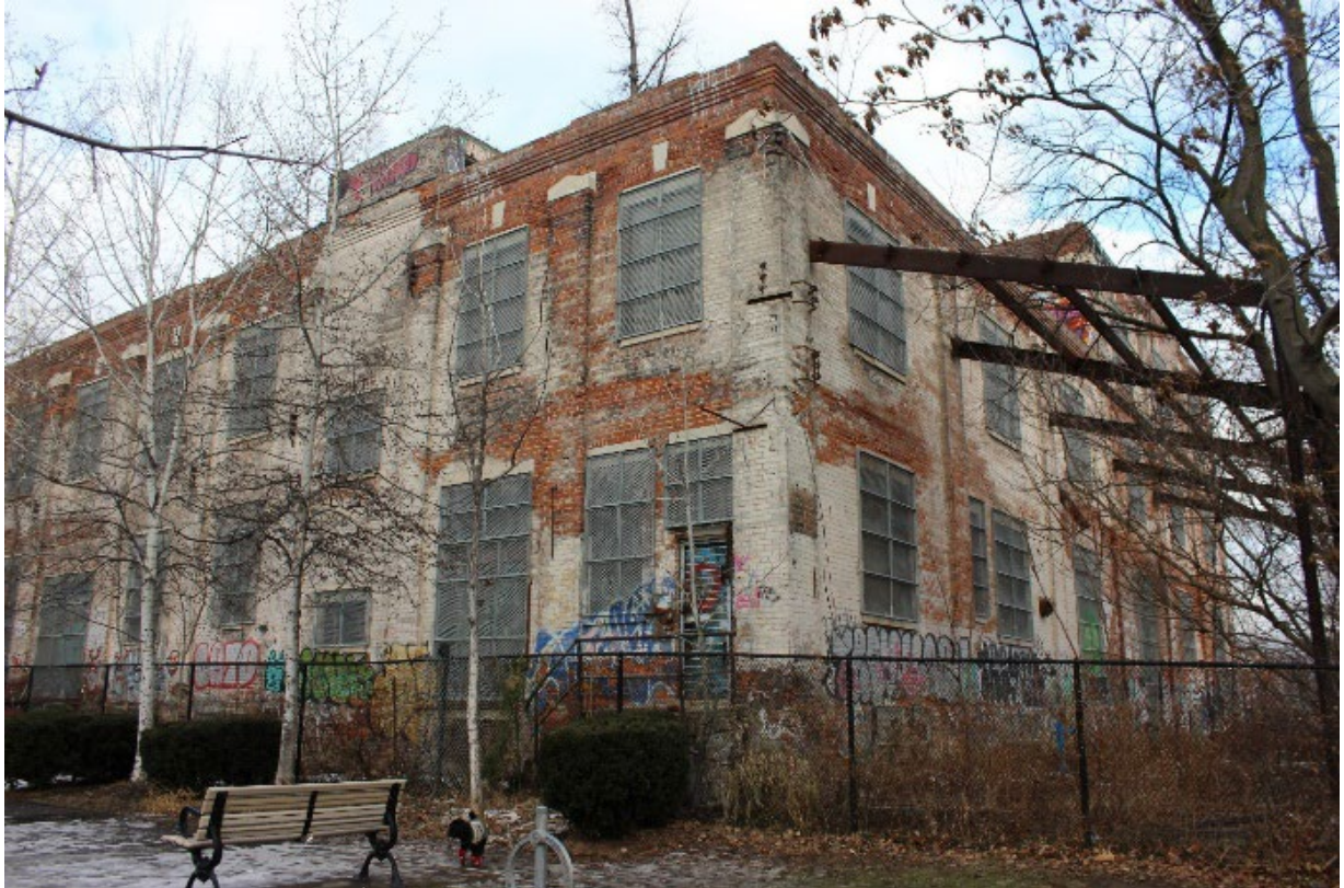
Figure 28. View of the southwest elevation with detail of the steel "lean-to" canopy frame (Heritage Planning, 2025).
