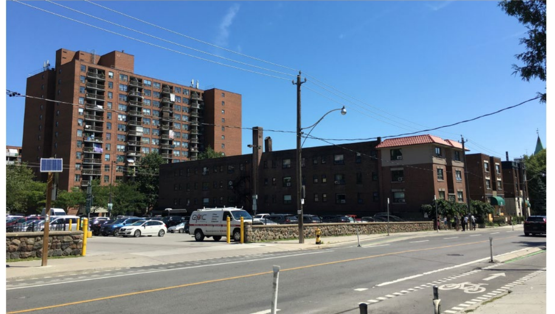
405 Sherbourne Street looking southeast (ERA Architects Inc., 2020)
