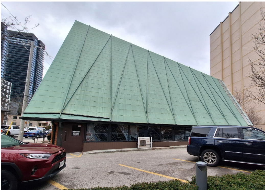
Figure 8 View of the south elevation of the Church Building. Note the copper clad roof with angled ridges (Heritage Planning, 2025).
