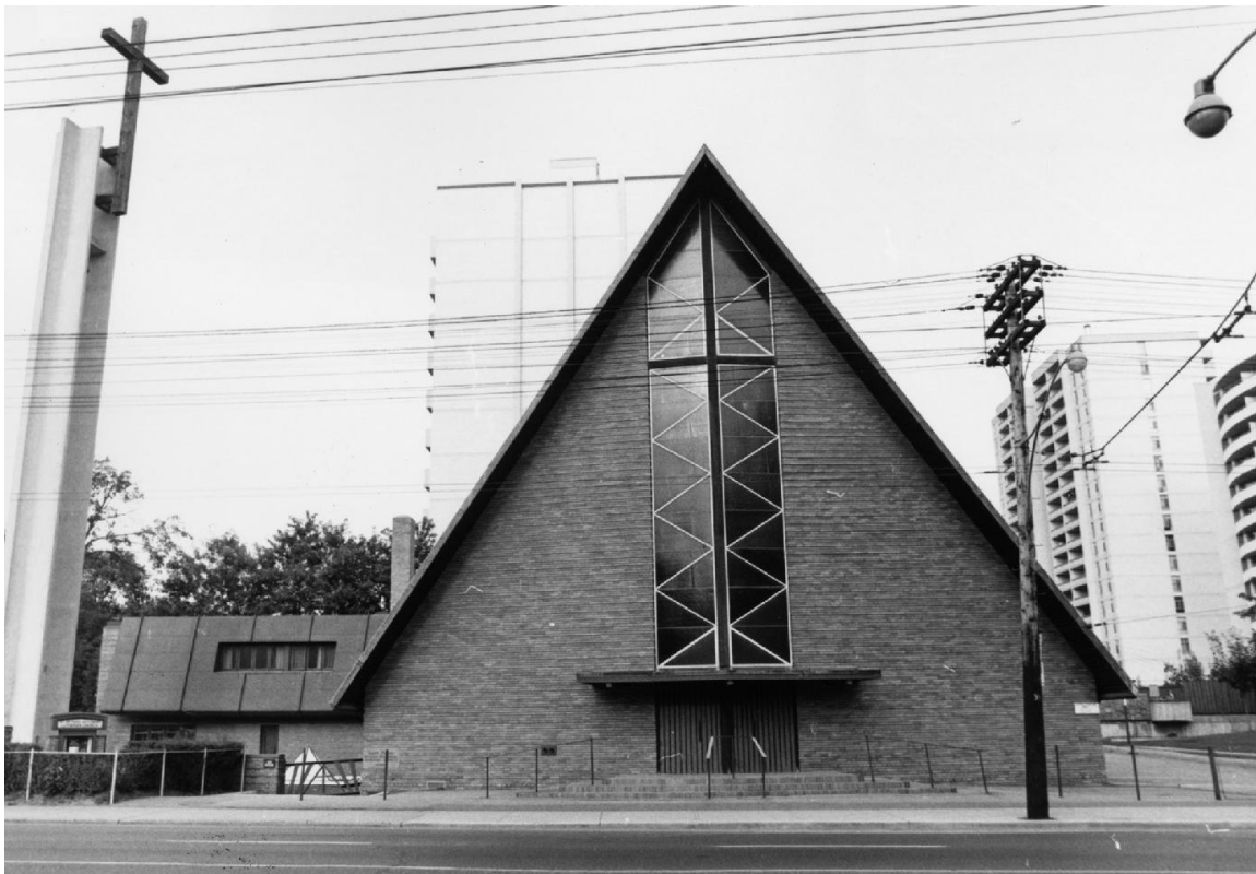
Figure 2 1981 image of the subject property from Mount Pleasant Road prior to the construction of the outer columbarium wall and removal of the cross from the bell tower (Toronto Archives).
