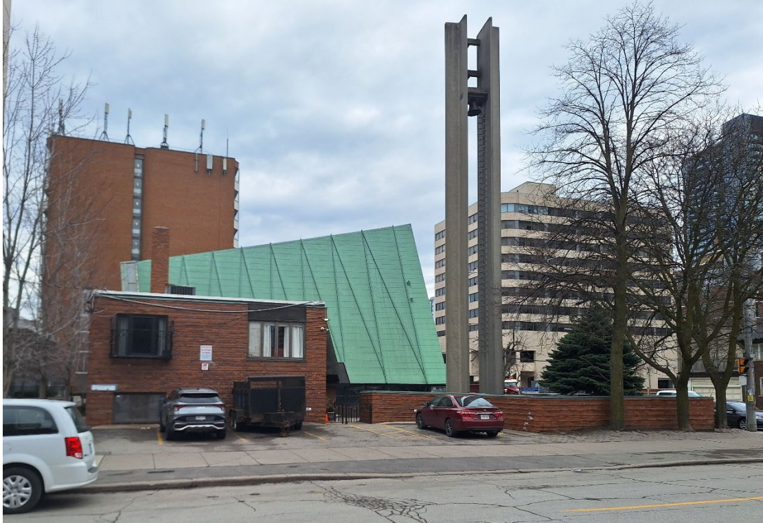
Figure 7 View looking south from Roehampton Avenue showing (left to right) the ancillary wing, Church Building, Bell Tower and Columbarium (Heritage Planning, 2025).
