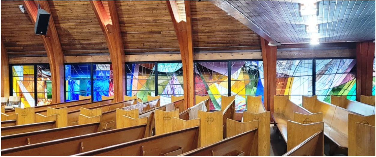
Figure 12 Interior view of south elevation showing coloured glass windows, glulam truss beams and pews (St. Peter's EELC, 2026).
