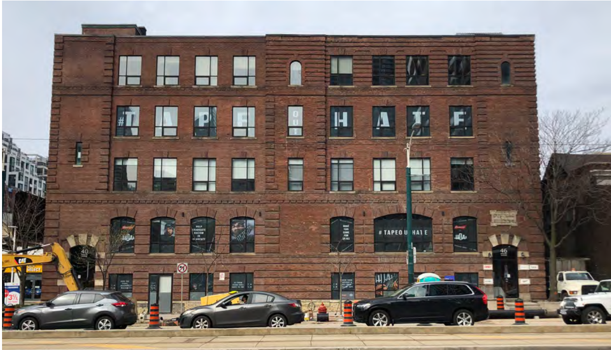
Figure 6. East elevation of 40-46 Spadina Ave (ERA, 2022).
