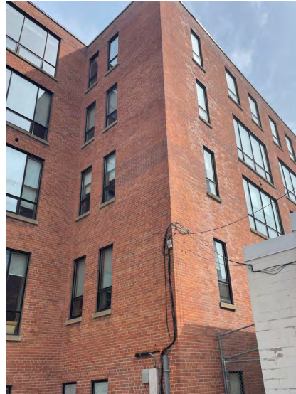
Figure 55. East portion of south elevation of 40-46 Spadina Ave (ERA, 2022).
