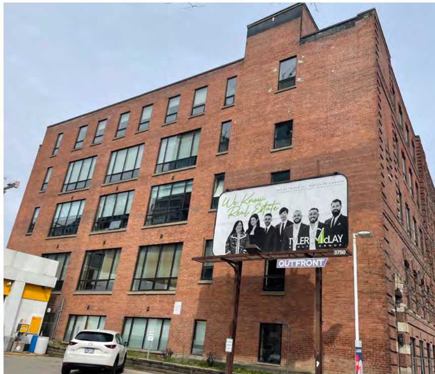
Figure 56. East portion of south elevation of 40-46 Spadina Ave (ERA, 2022).
