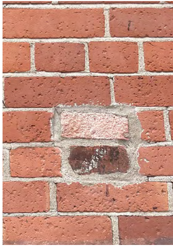
Figure 81. South elevation brick replacement (ERA, 2022).
