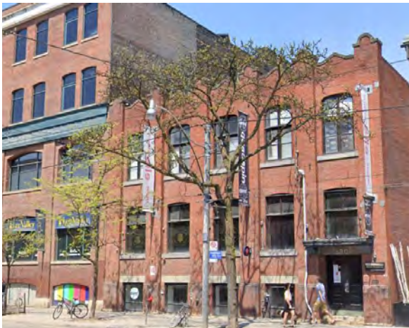
Figure 36. Warehouse and factory located at King and Portland Street, constructed in 1904 (Google Street View, 2021).
