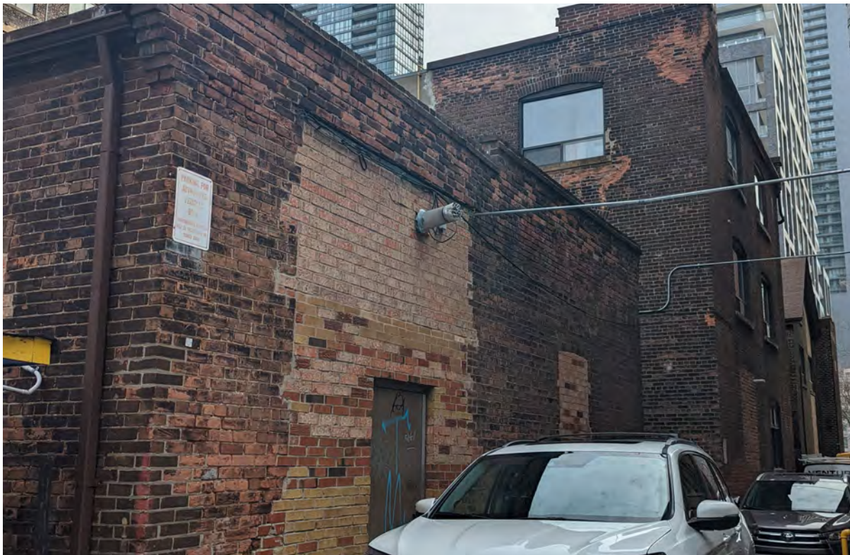
Figure 15. South elevation of rear structures (ERA, 2022).
