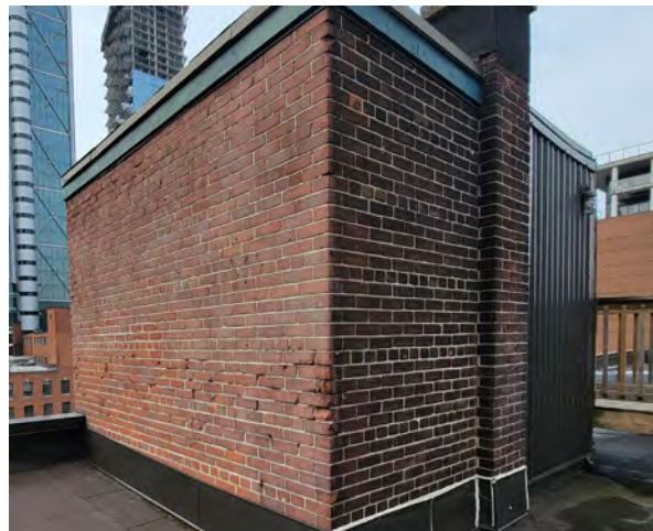
Figure 90. Main elevator shaft (ERA, 2022).
