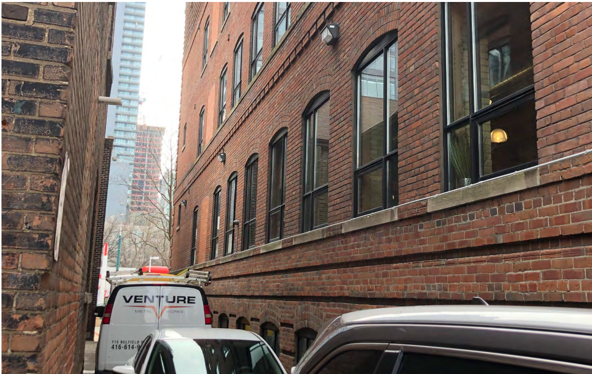
Figure 9. North elevation of 40-46 Spadina Ave looking east (ERA, 2022).
