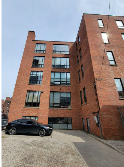
Figure 54. West portion of south elevation of 40-46 Spadina Ave (ERA, 2022).
