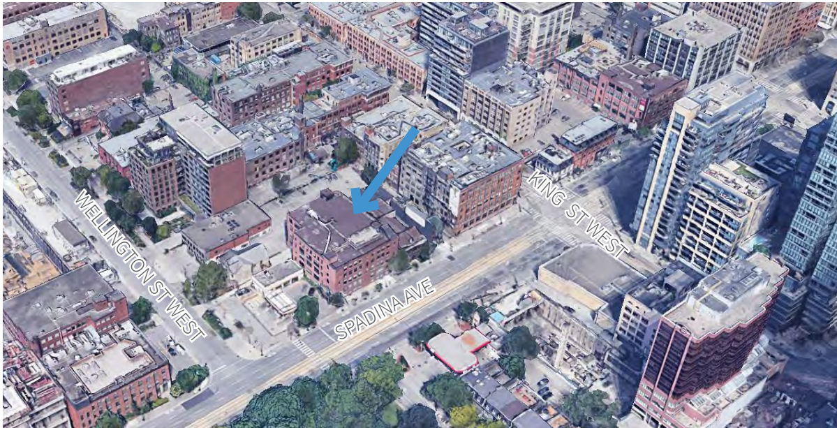
Figure 18. View of the Site showing the surrounding context (Google Earth 2019; annotated by ERA)
