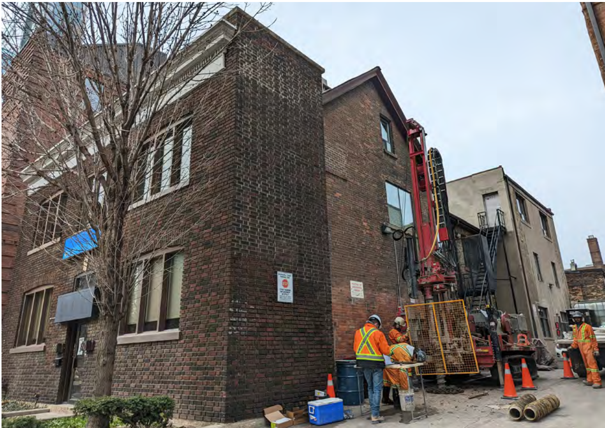
Figure 12. East and north elevations of 58-60 Spadina Ave (ERA, 2022).
