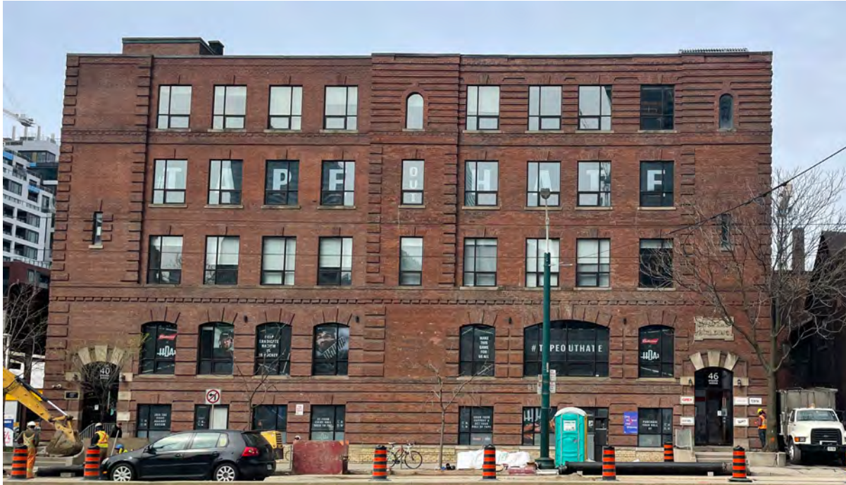
Figure 49. East elevation of 40-46 Spadina Ave (ERA, 2022).
