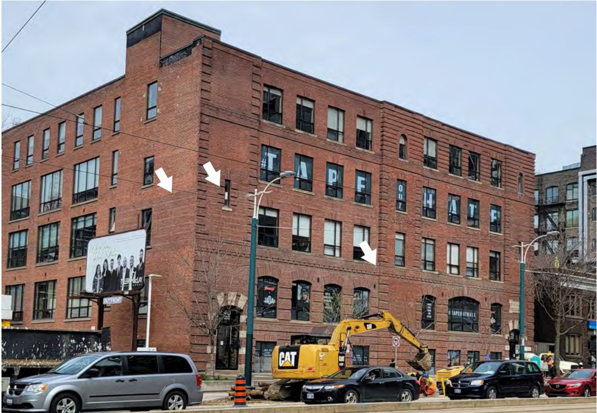
Figure 66. East elevation of 40-46 Spadina Ave with arrows indicating changes in brick colour (ERA, 2022).
