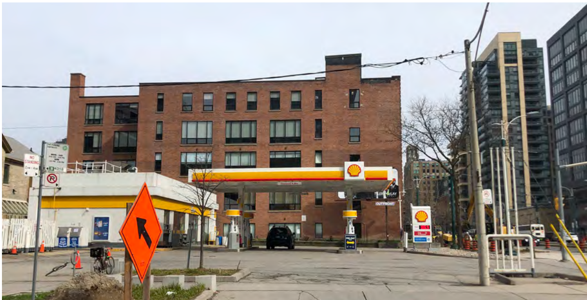
Figure 7. South elevation of 40-46 Spadina Ave (ERA, 2022).
