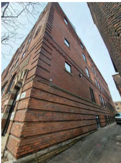
Figure 50. North elevation of 40-46 Spadina Ave viewed from laneway (ERA, 2022).
