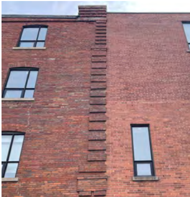
Figure 71. The west elevation changes in brick (ERA, 2022).
