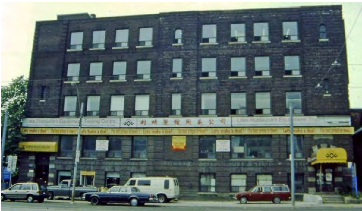
Figure 24. The east elevation of the Site (City of Toronto, 1999).
