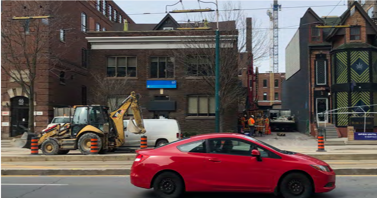
Figure 10. East elevation of 58-60 Spadina Ave (ERA, 2022).
