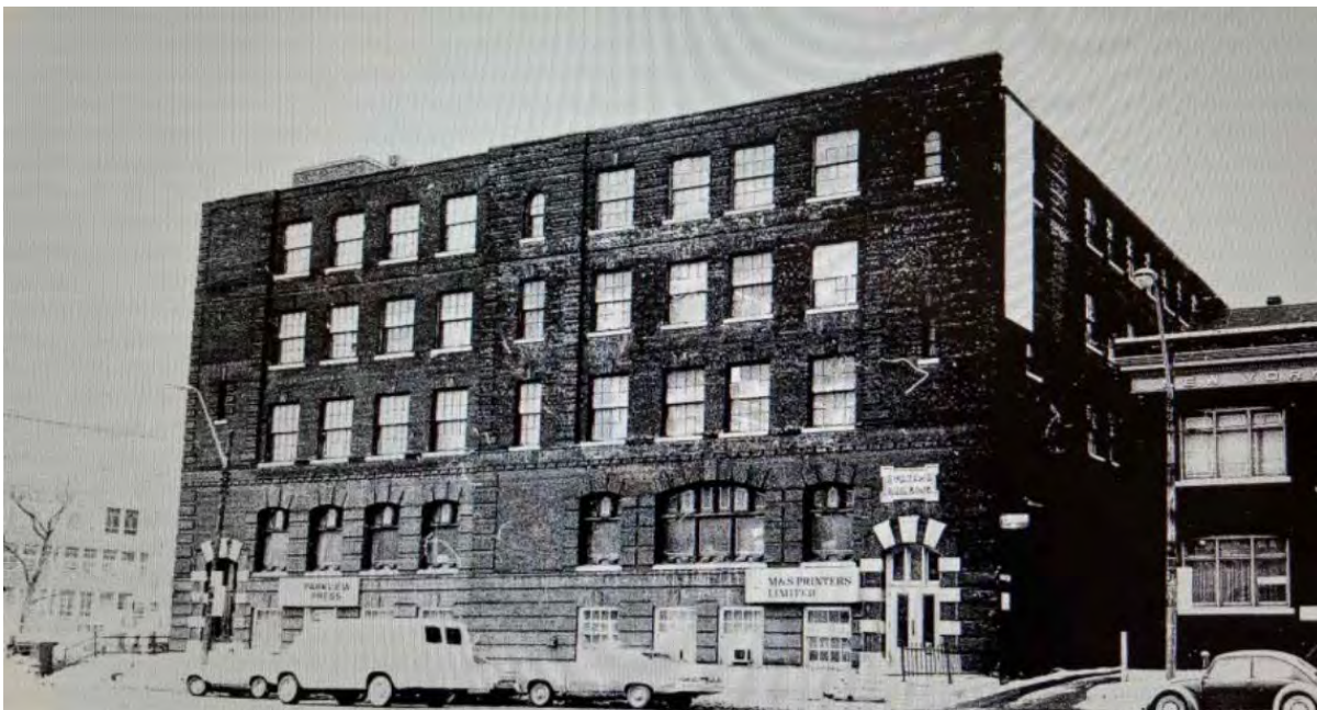
Figure 22. The east elevation of the Site (City of Toronto, 1975).
