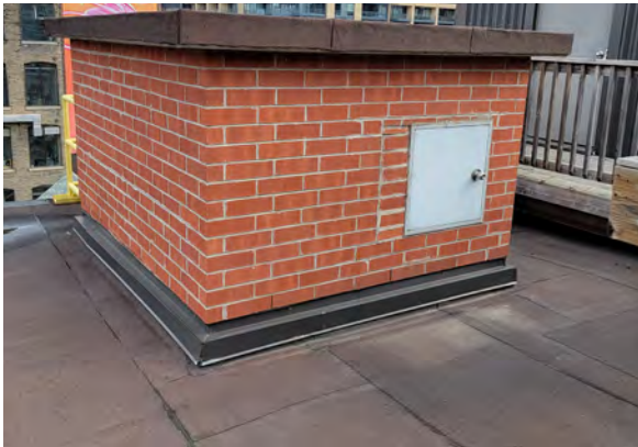
Figure 87. North elevator shaft at rooftop (ERA, 2022).
