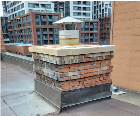
Figure 89. West central chimney (ERA, 2022).
