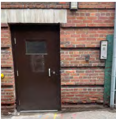
Figure 103. Steel door for maintenance access at north elevation (ERA, 2022).
