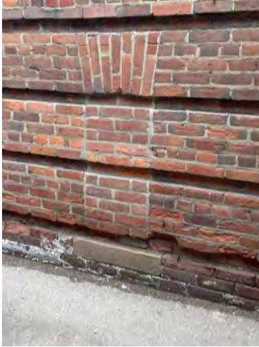
Figure 104. Basement window infill at north elevation (ERA, 2022).
