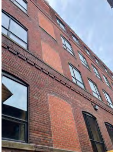
Figure 105. Second bay from east side of the north elevation displaying window infill (ERA, 2022).
