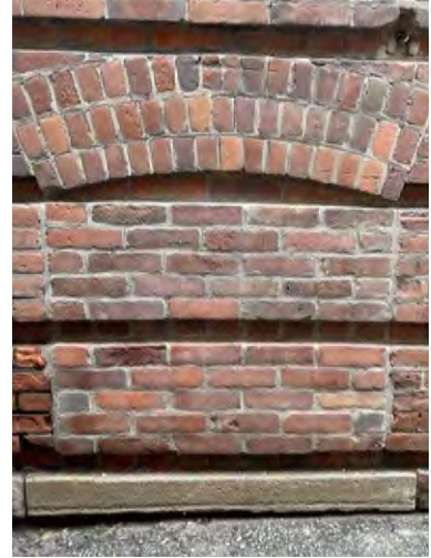
Figure 106. Basement window infill at north elevation (ERA, 2022).
