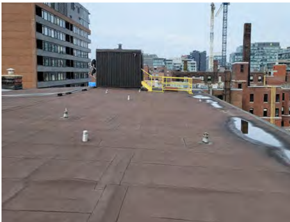
Figure 109. Built up roof system with membrane (ERA, 2022).
