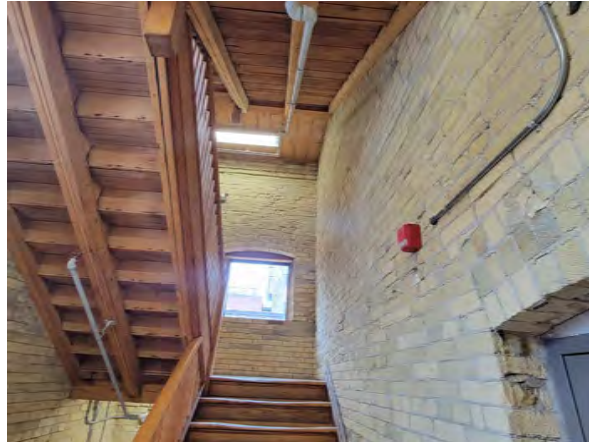
Figure 113. North east stairwell (ERA, 2022).
