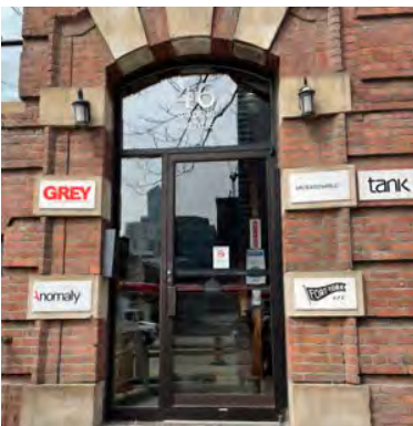
Figure 102. Typical door condition at east elevation (ERA, 2022).
