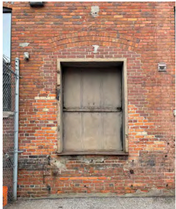
Figure 108. Maintenance door opening at west elevation displaying several surrounding brick replacements (ERA, 2022).
