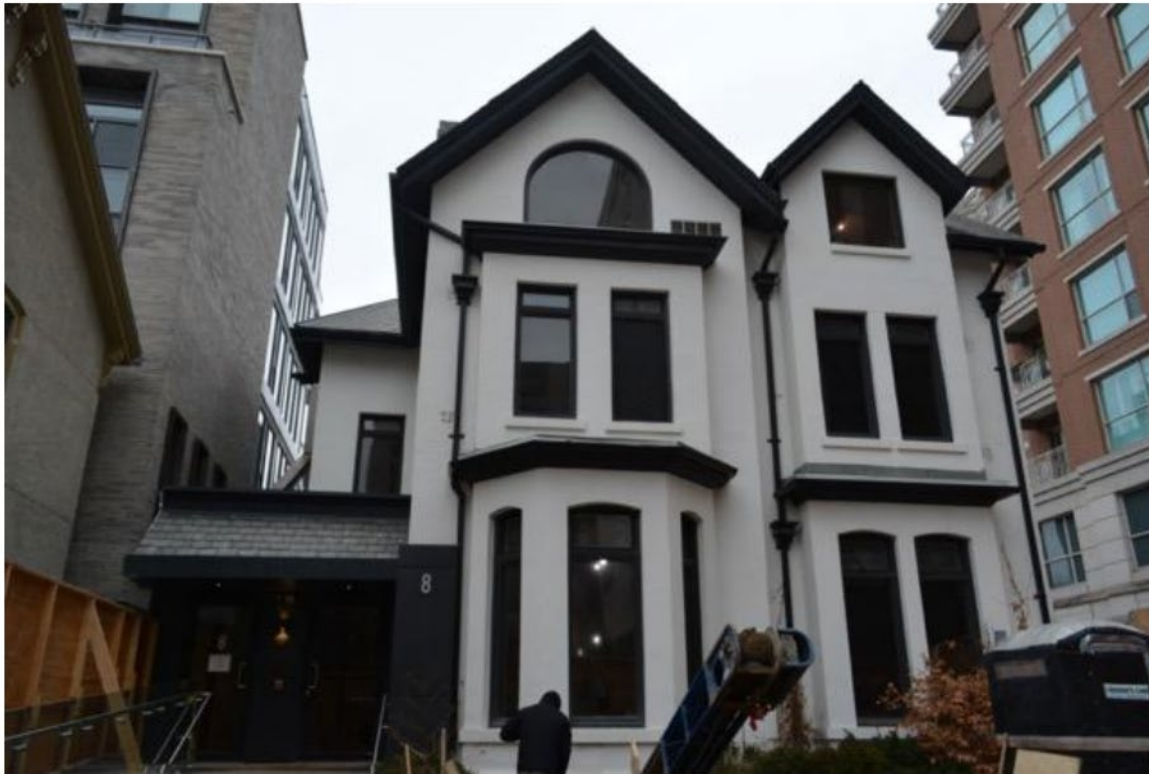
Primary (south) elevation of 8 Prince Arthur Avenue showing the building as seen from Prince Arthur Avenue. The entrance with the sloped roof on the left is proposed to be replaced with a flat roof. Partial view of the property at 10-14 Prince Arthur Avenue is seen on the left (Source: GBCA Architects, 2026)
