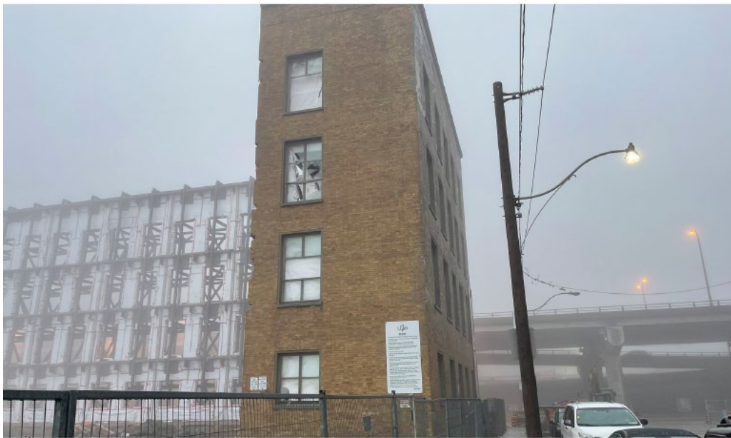
Figure 10: South and east elevation of the Office Building, looking north (Giaino + Associates Architects Inc., 2026).
