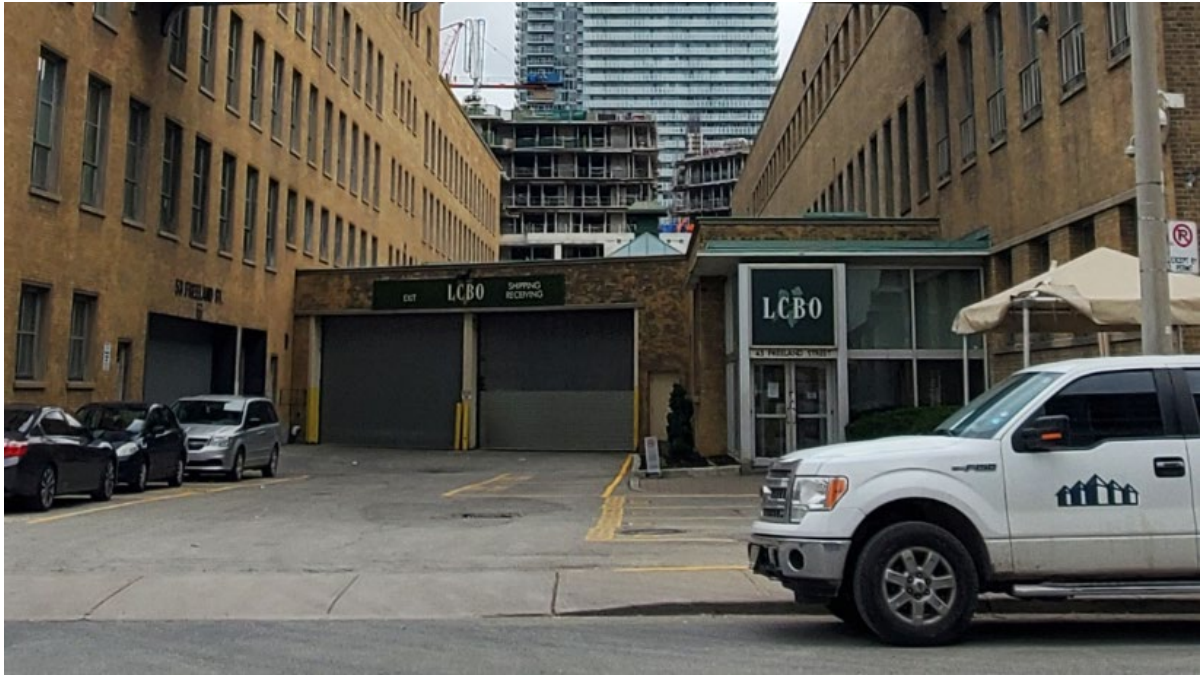
Figure 7: Detail of the side (west) entrance to the Warehouse Building and the rolling garages in the one-storey connecting building (Heritage Planning, 2020)
