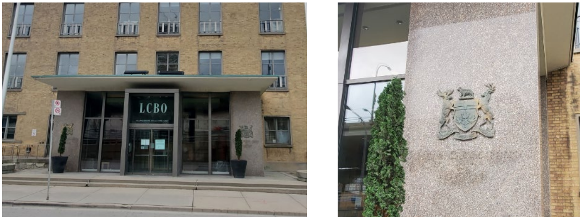
Figure 3a and 3b: Detail of the main entrance in the principal (north) elevation of the Office Building (left) and one of the "Province of Ontario" crests (right) (Heritage Planning, 2020)
