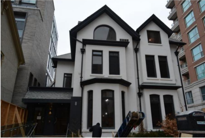
Primary (south) elevation of 8 Prince Arthur Avenue showing the building as seen from Prince Arthur Avenue. (Source: GCBA Architects Inc., 2026;)
