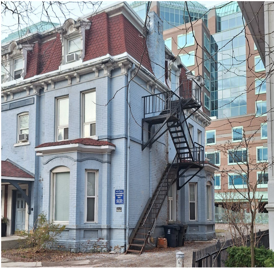
Figure 9 Looking southwest toward north elevation of 40 Huntley Street (Heritage Planning, 2026).
