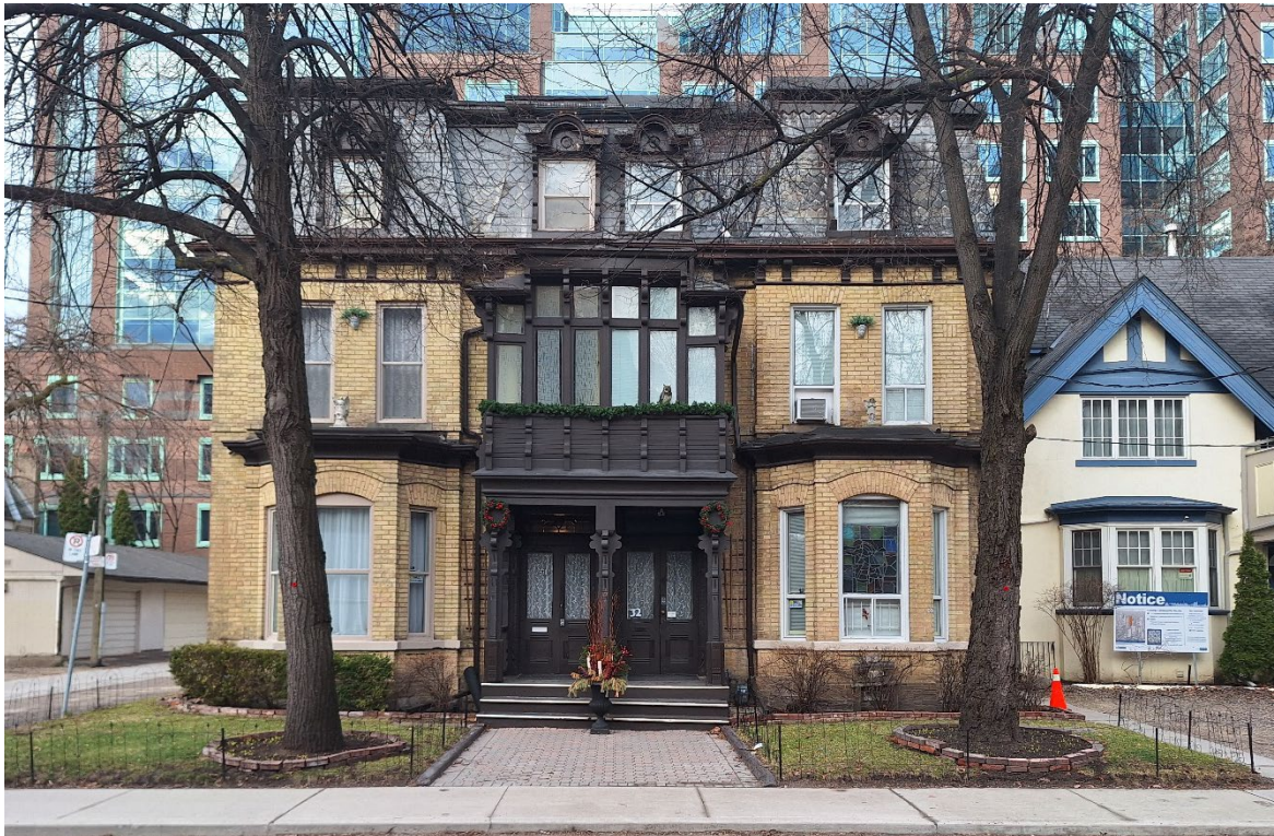
Figure 2 Principal (east) elevation of 30 and 32 Huntley Street (Heritage Planning, 2026).
