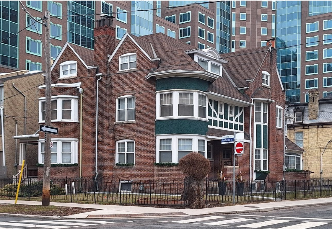
Figure 12 View looking northwest towards the principal (south) elevation of 122 and 124 Isabella Street and east elevation of 124 Isabella Street (Heritage planning, 2026).
