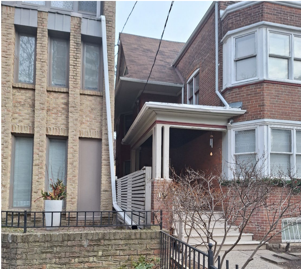
Figure 14 Partial view of west elevation of 122 Isabella Street showing entrance porch and gabled bay (Heritage Planning, 2026).
