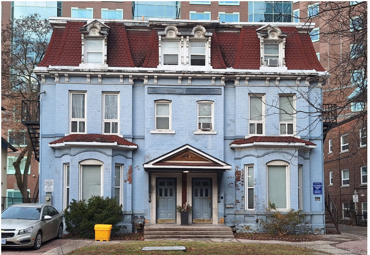
Figure 8 Principal (east) elevation of 38 and 40 Huntley Street, Heritage Planning, 2026).
