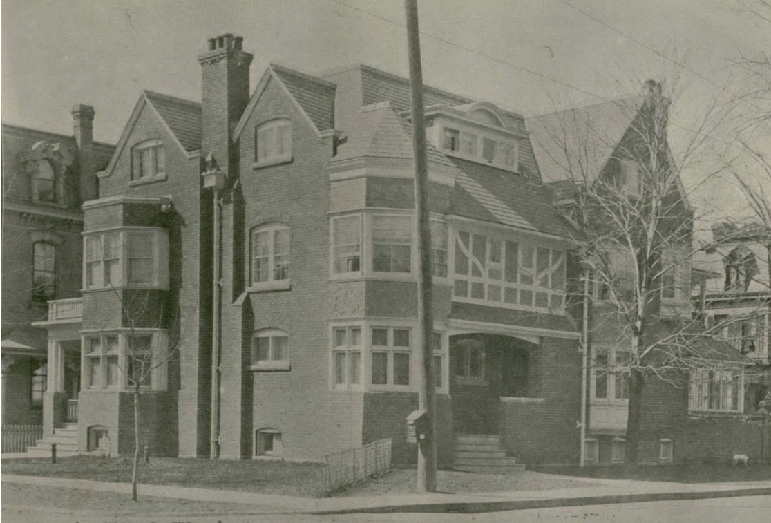
Figure 11 1902 image looking northwest towards the principal (south) elevation of 122 and 124 Isabella Street and east elevation of 124 Isabella Street (The Canadian Architect and Builder, 1902)
