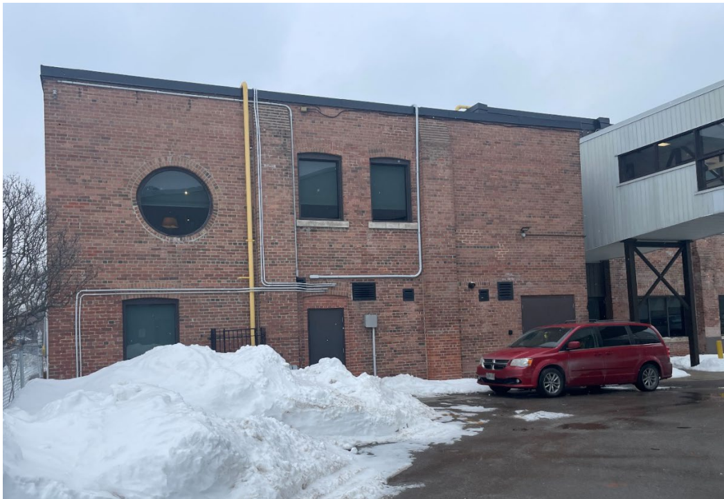
Figure 21. View of the south elevation of the south wing which features a circular window on the second storey and a segmental arch window opening at the first storey (Heritage Planning, 2026).
