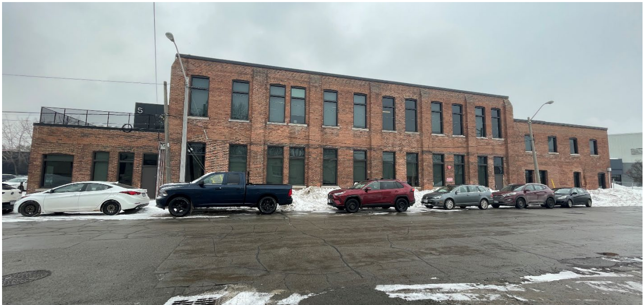
Figure 18. View of the west elevation of the west building, the Office and Aqua Ammonia Building, showing the central building in the middle, one storey north wing to the north, and the two storey south wing to the south (Heritage Planning, 2026).
