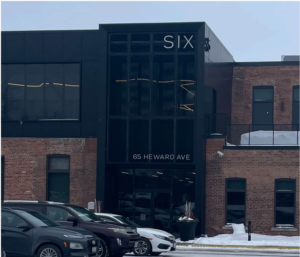
Figure 26. View of the north elevation of the Central Addition, originally constructed in 1987 and modified as part of the second storey addition to the Storage and Anhydrous Ammonia Building in 2019, featuring a steel and glass clad north elevation with double entrance at the first storey.
