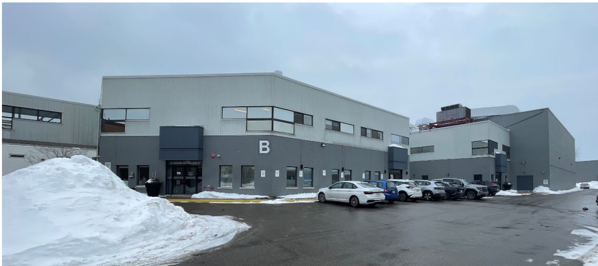
Figure 27. View of the north and west elevations of Studio Building, constructed to house film and television studios, featuring rectangular windows.
