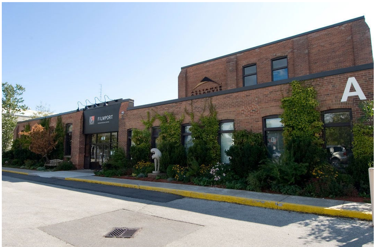
Figure 15. 2008 image showing the principal (north) elevation, where the two buildings dating from 1913 were merged into a single structure as a part of the 1987 redevelopment (CTA).
