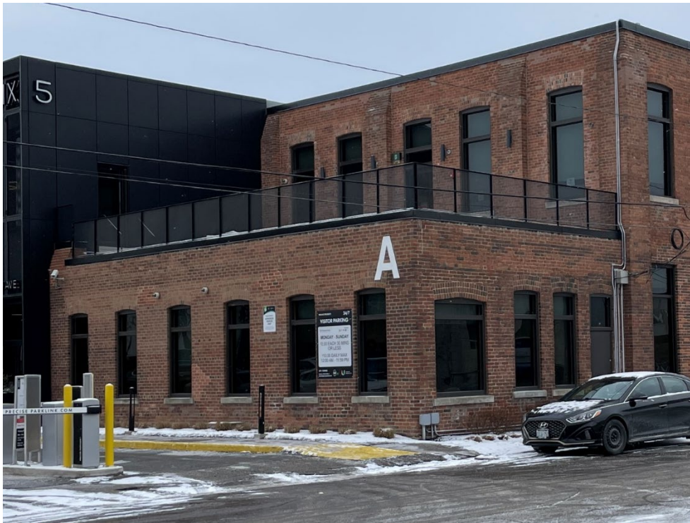
Figure 22. View of the north and west elevations of the one-storey north wing of the Office and Aqua Ammonia Building, featuring segmental arched window and door openings with brick voussoirs (Heritage Planning, 2025).
