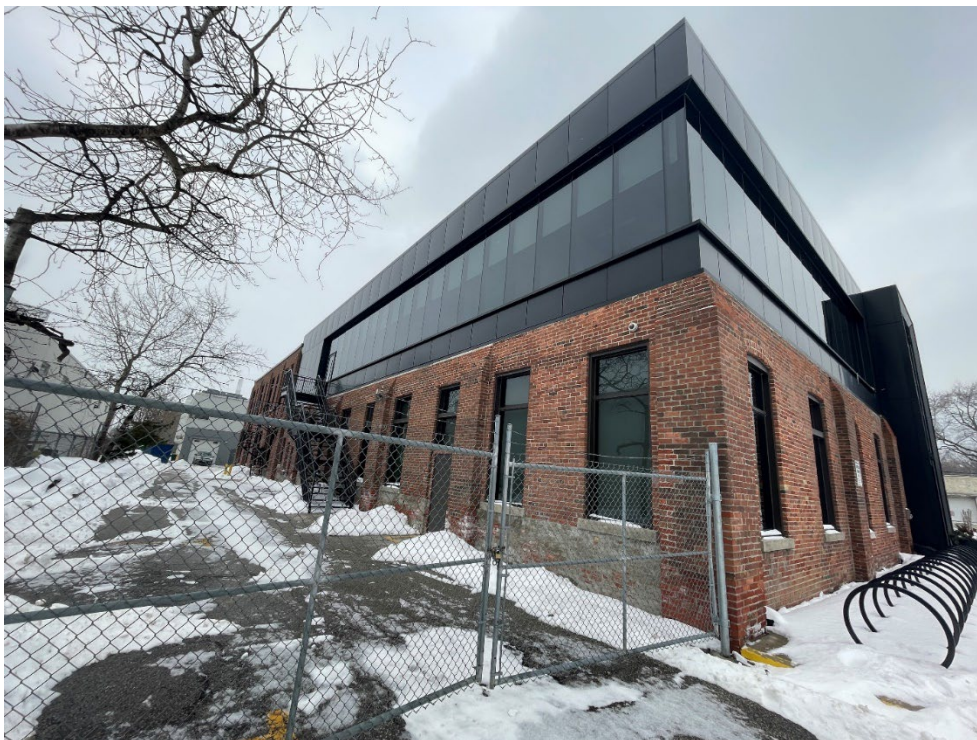
Figure 23. Partial view of the north and east elevations of the Storage and Anhydrous Ammonia Building featuring the one-storey north section with a second storey glass clad addition from 2019 (Heritage Planning, 2026).
