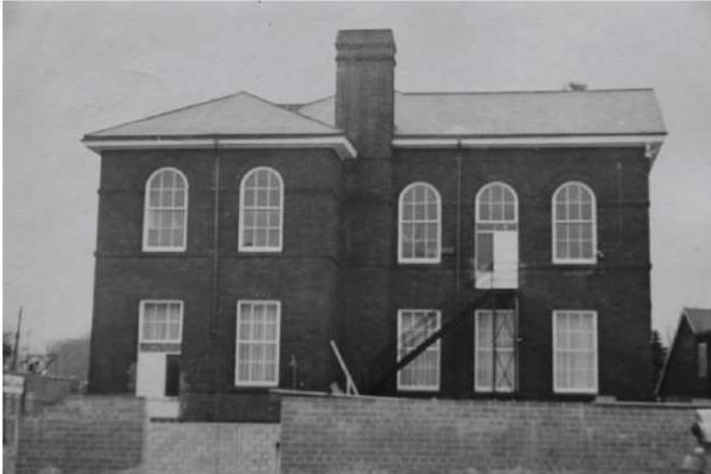
Rear (west) elevation of 1891 schoolhouse in early 1960s. 1963 addition under construction in the foreground (Estonian House, year unknown).
