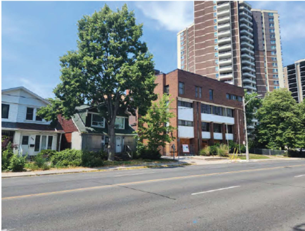
Updated view looking northwest toward the site (ERA, 2025).
