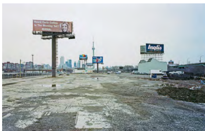
Figure 25: Former Inglis lands following demolition, looking east towards Strachan Avenue, 2002 (Peter MacCallum, courtesy of Toronto Public Library).
