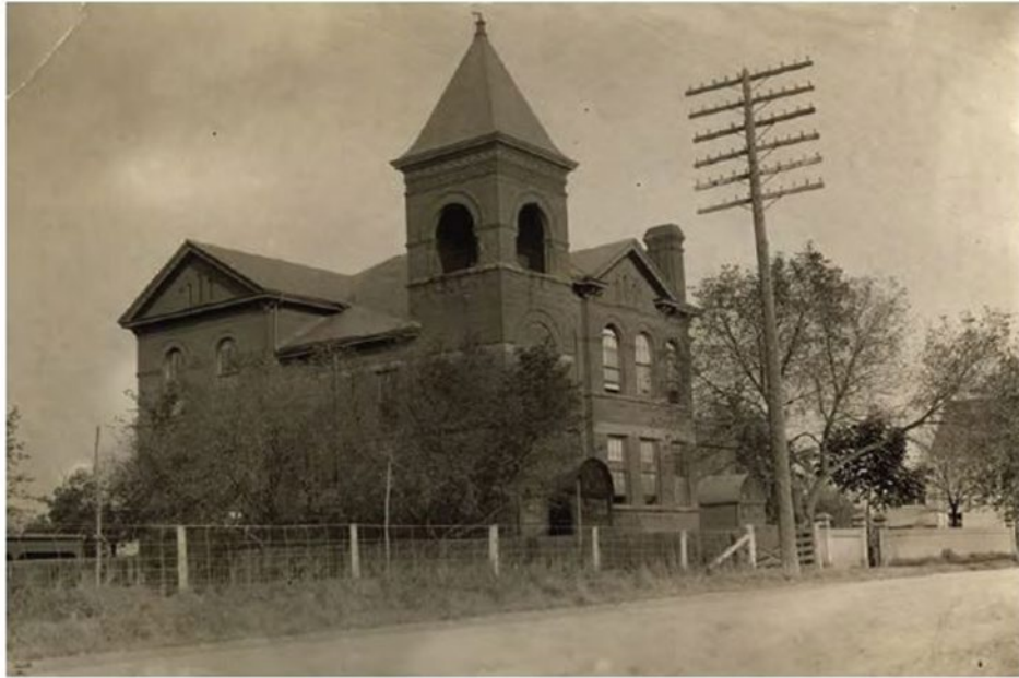
Looking north-west towards the subject site, 1905 (Toronto Public Library).
